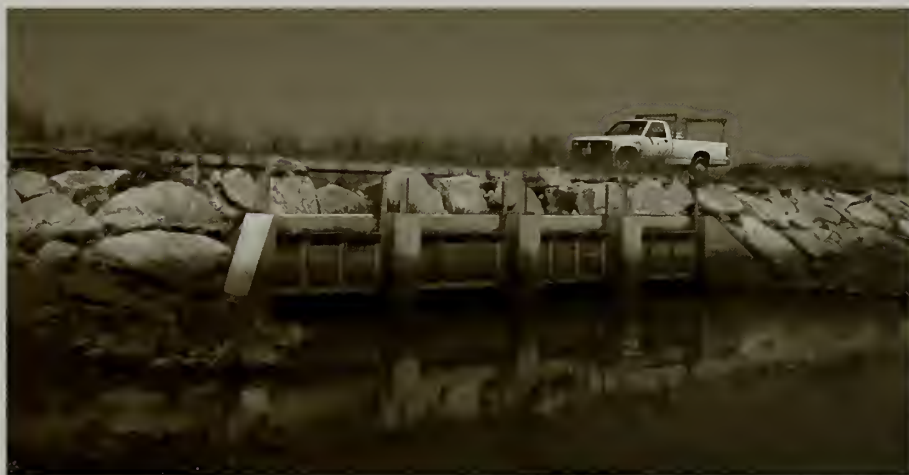
Figures 3 (photo) and 4 (graph). In 1997, a planning and regulatory team with members from local, state, and federal agencies approved a culvert configuration and general restoration plan for Hatches Harbor. The installation of new culverts occurred in January 1999, following two years of pre-restoration monitoring. The photograph shows four new 7-foot-wide-by-3-foot-high culverts at Hatches Harbor with adjustable tide gates that are about half open. The graph documents how tidal range has increased in diked portions of the Hatches Harbor salt marsh with the installation and incremental opening of large culverts. Numbers above bars are cross-sectional areas (m 2 ) of culvert openings.
