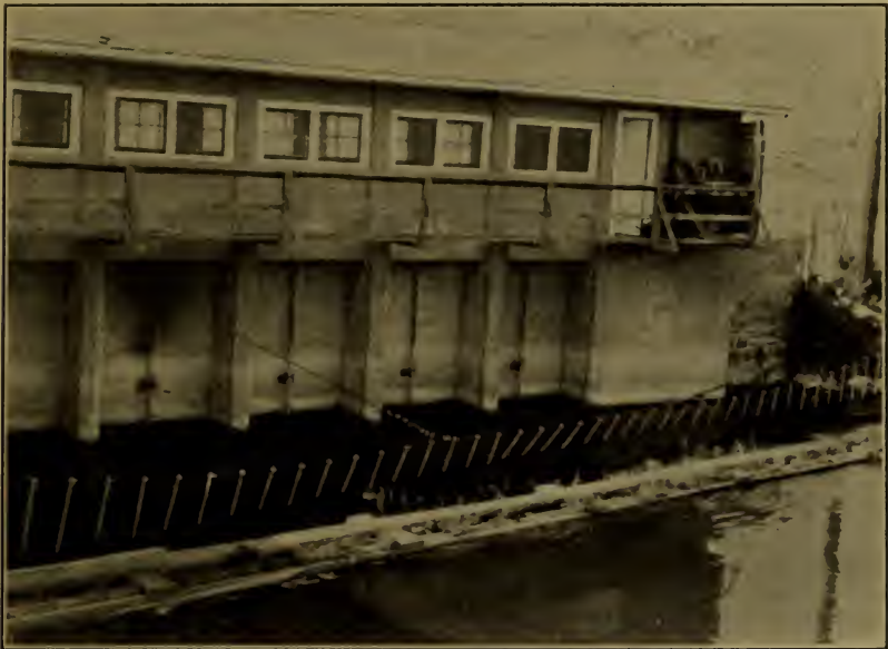
FIGURE 6.—The Wapato electric fish screen. Chain electrodes are seen hanging in front of the diversion gates
