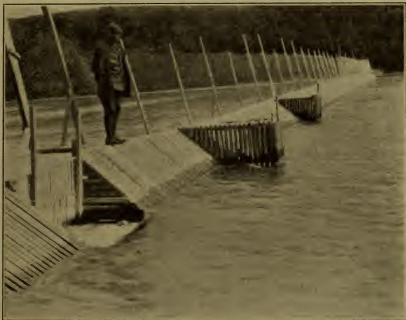
FIGURE 5.—A salmon counting weir in Alaska. Enumerators count each fish that passes through the opening shown in the foreground
