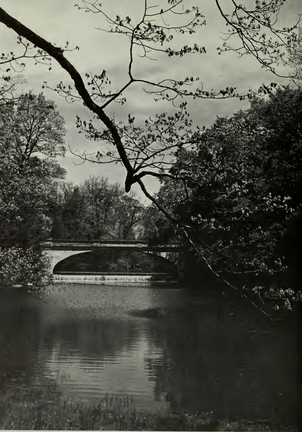
White Bridge from the south.
