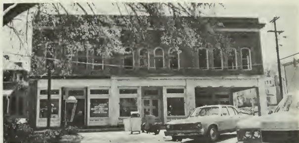
Fig. 1. Abbeville Town Square. Storefronts, south facade, before project work. May 1978. Photo: Stuart Johnson.
