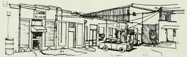
Fig. 19. Abbeville Town Square. Existing conditions behind block of shops in the commercial square. Sketch: Triad Architectural Associates, Architects.
