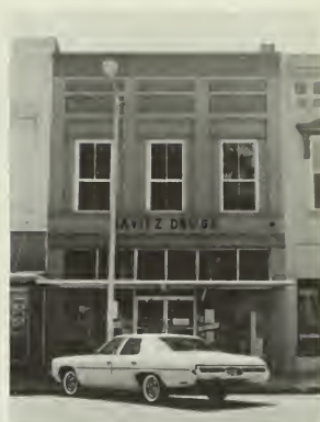
Fig. 7. Abbeville Town Square. Storefront, west facade, after project work has been completed. February 1979. Photo: Stuart Johnson.
