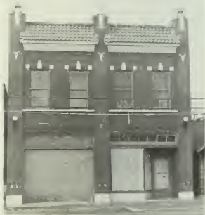
Fig. 5. Abbeville Town Square. Storefront, west facade. Publicly-owned Abbeville Fire Station, after project work has begun. March 1979. Photo: Stuart Johnson.
