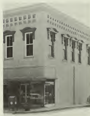
Fig. 9. Abbeville Town Square. Storefront, southwest facade, after project work has been completed. February 1979. Photo: Stuart Johnson.
