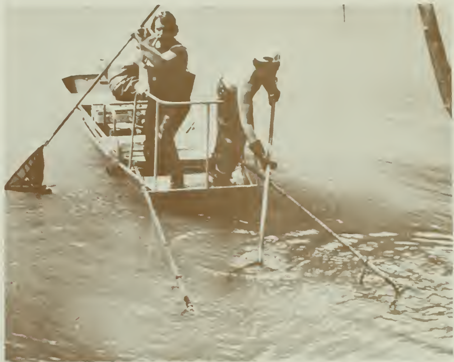
Sampling for fish with an electro-shocker in the tailwater below Green River Lake, Kentucky. Fish are collected with nets after they are drawn to the surface by the current.
