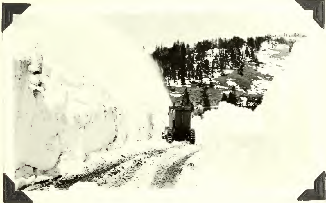
Sno-go rotary snow plow clearing Dunraven Pass about one-quarter mile south of pass. Snow 12 feet deep just behind plow. Picture taken May 24, 1933.
