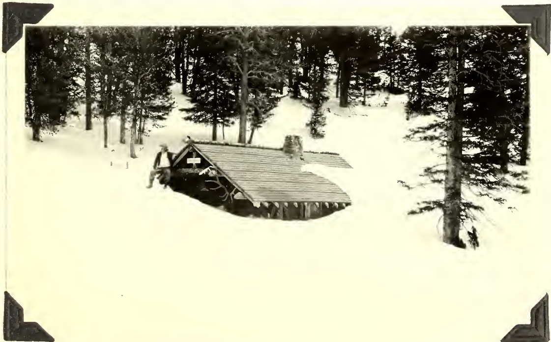
Dunraven Pass ranger station on May 24, 1933
