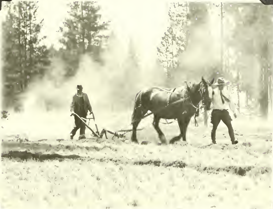
Showing the use of a plow for building fire trench on the West Yellowstone fire, May 30, 1935.
