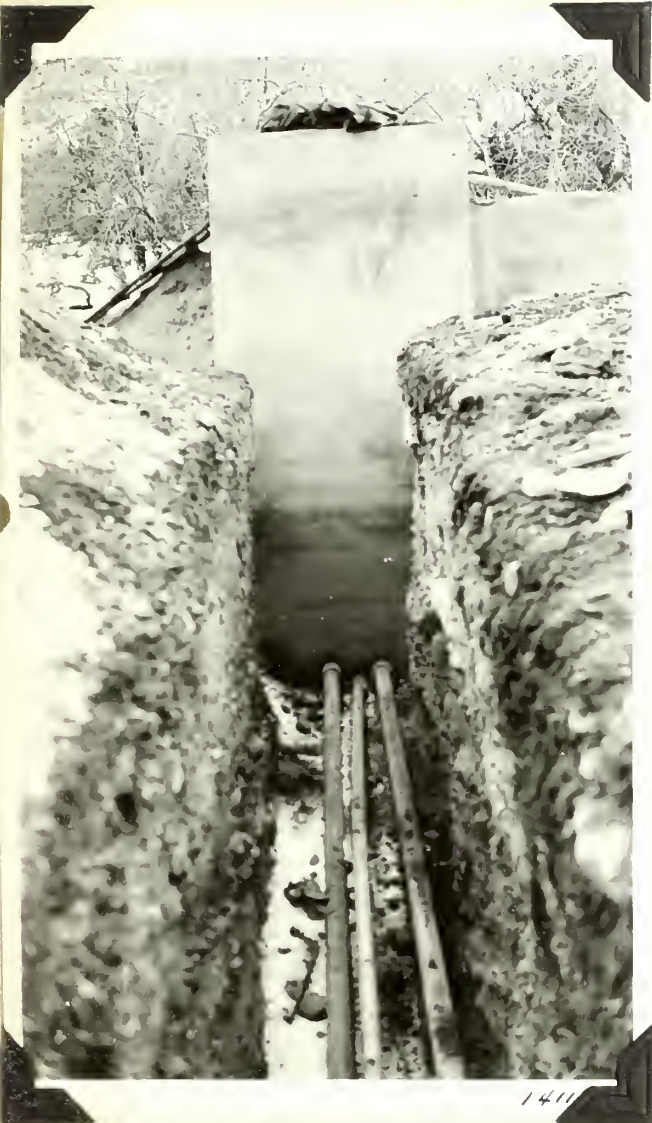
(at right) Pipe line laid by unrollies at New Ranch during fourth period. Pipe line (on left) is blow-off; center is unhole drain; and one on bottom of ditch is the main line.
