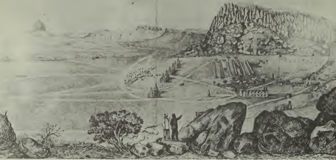
Fort Davis in October 1867, as it is being constructed. The view is from the slope north of the post. In the center are the roofless shells of the old stone barracks built in 1856 by Colonel Seawell. At the right are the scattered ruins of the first fort and the camp of the 9th Cavalry; between the rows of tents are temporary stables made of poles and thatched roofs. To the left of the barracks, work is beginning on officers' row.
