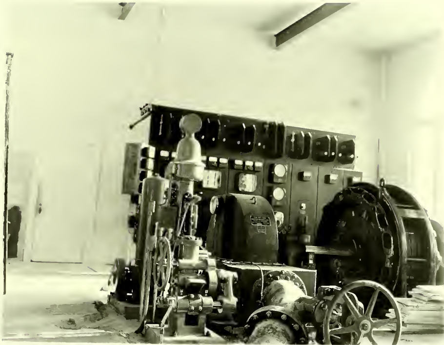
11276-1 (1936) Water & Power Development, Mammoth. Project F.P. 598. View of Woodward governor, water wheels, generator and switchboard in background.
