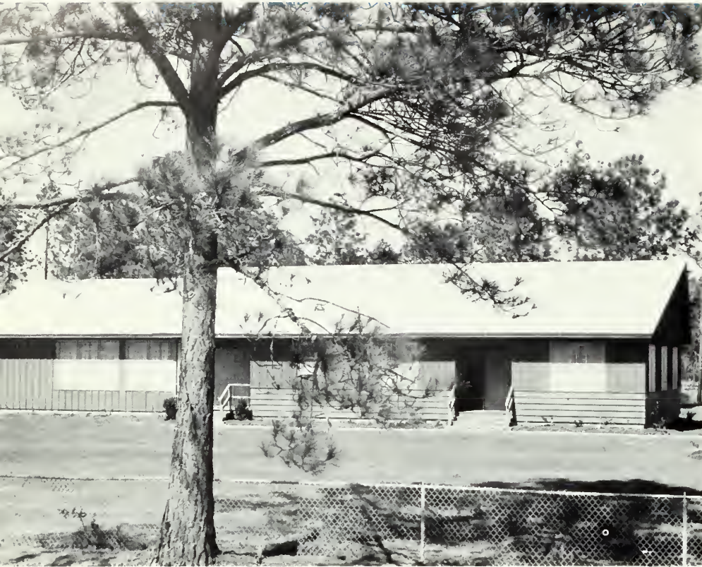
The Charles H. Herty Building is headquarters for the Waycross State Forest.
