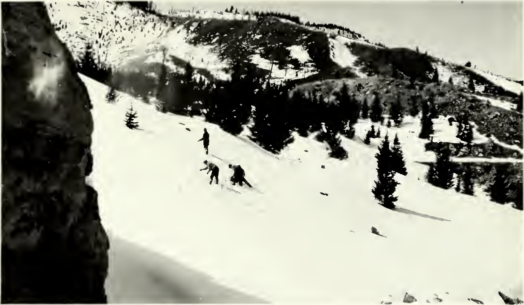
Taken April 7, 1932. Opening the road near the Hoodoos. Placing powder for blowing out drift.
