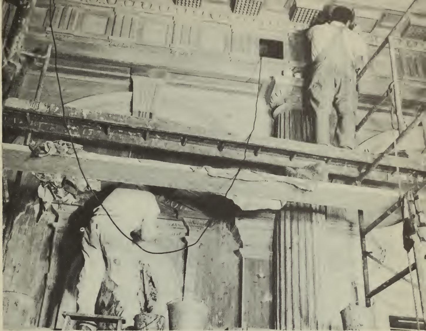
Architectural investigation in Independence Hall, 1956. Above: Removal of paint and restoration of woodwork. Below: Detail of hand-carved decoration after paint removal.
