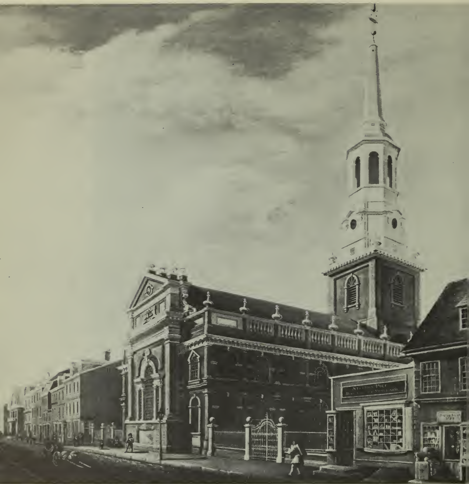
Christ Church (built 1727–54) where George Washington, Benjamin Franklin, and other notables worshiped; seven signers of the Declaration of Independence are buried in its grounds and cemetery. Painting by William Strickland, 1811. Courtesy Historical Society of Pennsylvania.
