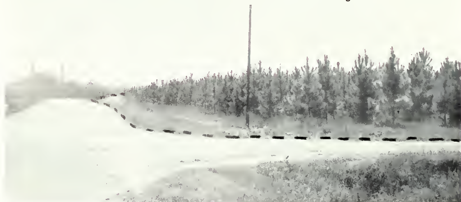
Plant Building Site
