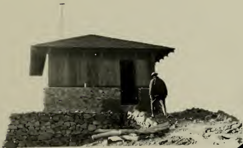
Project 831 - Lookout at Mt. Sheridan. Windows boarded up for winter.
