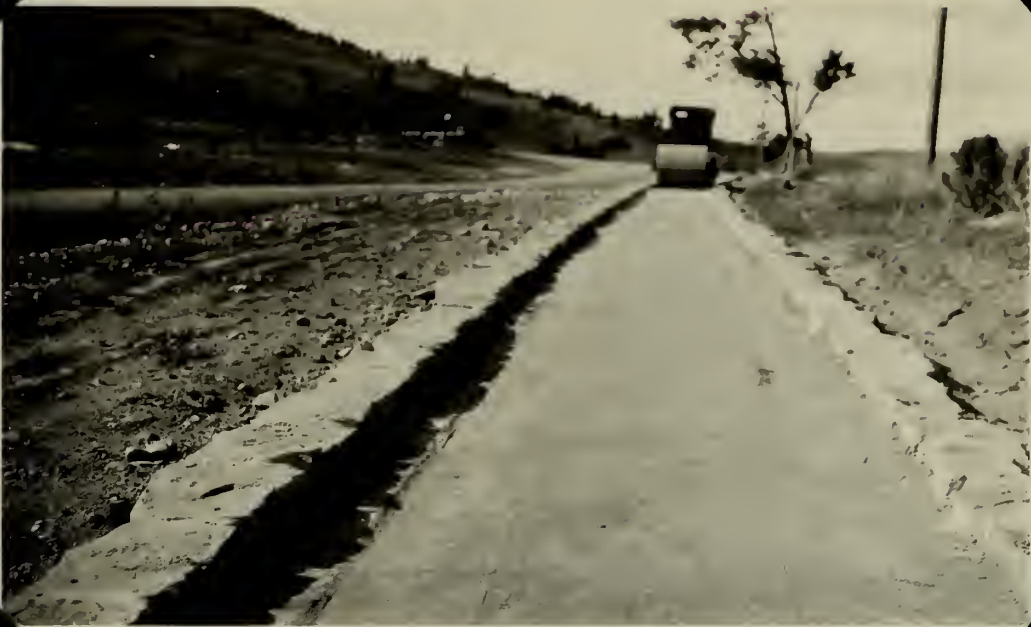
Project 502.26 Sidewalk at Mammoth. Sub-grade rolled, ready for gravel.
