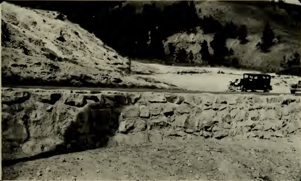
Project 502.26 - Sidewalk at Mammoth. Showing new stone wall.
