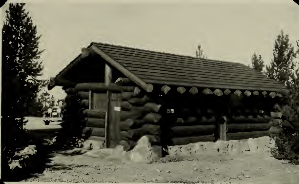
Project 421 - Comfort station at Norris. Shows completed structure except for gable window. Since completed.
