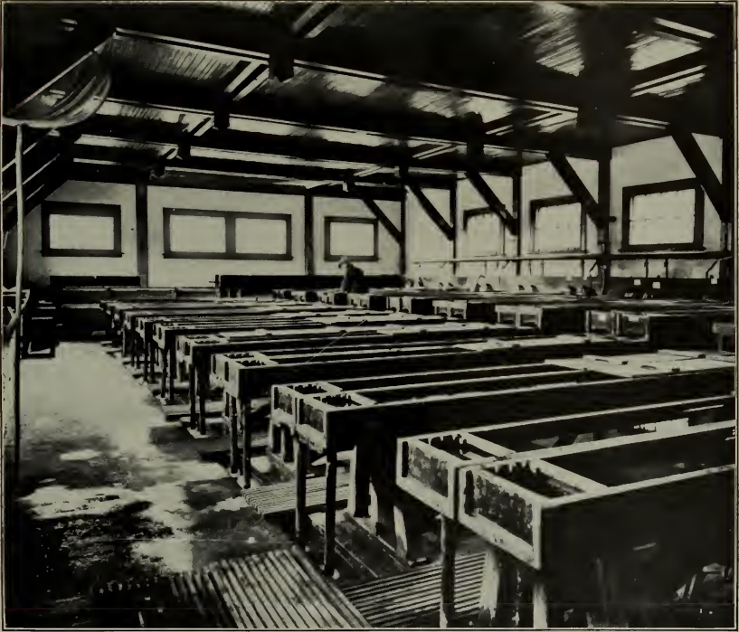
FIG. 5.—Interior of St. Johnsbury (Vt.) station.
