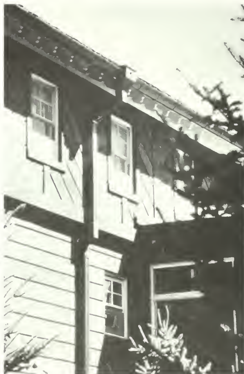
Sun Valley Lodge, Idaho – Form Board Concrete Walls
