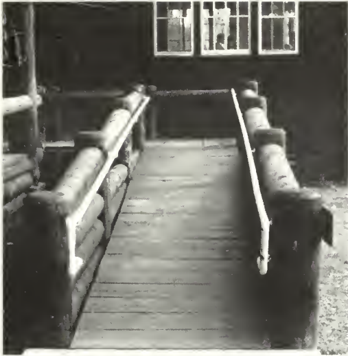
Handicap Ramp at Yellowstone National Park
