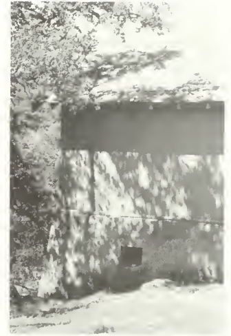
Utility Building at Ash Mountain
