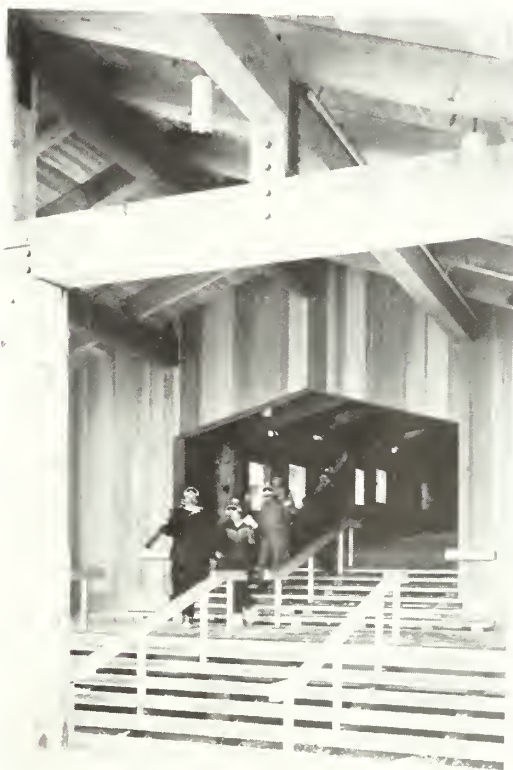
Covered Entry at Snow Park Lodge, Deer Valley
