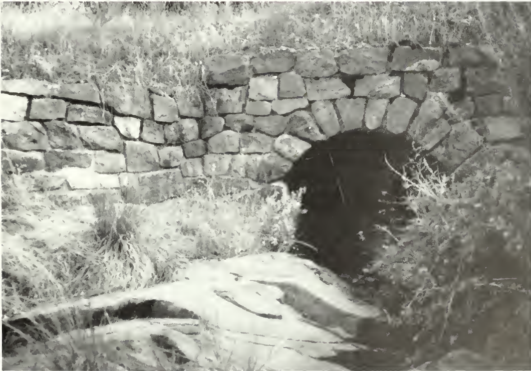
Stone Culvert in Sequoia National Park
