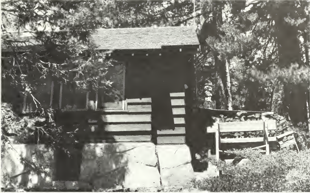
Grant Grove Ranger Residence
