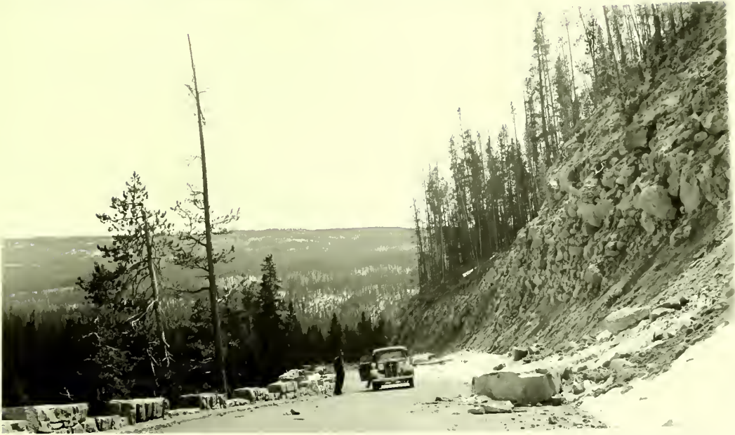
Rock slide at Gibbon Canyon with indication of more to come.
