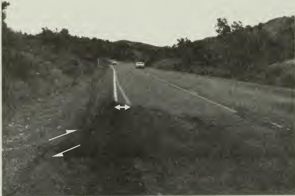
Figure 8.--Displacement of pavement by Coal Hill landslide.
