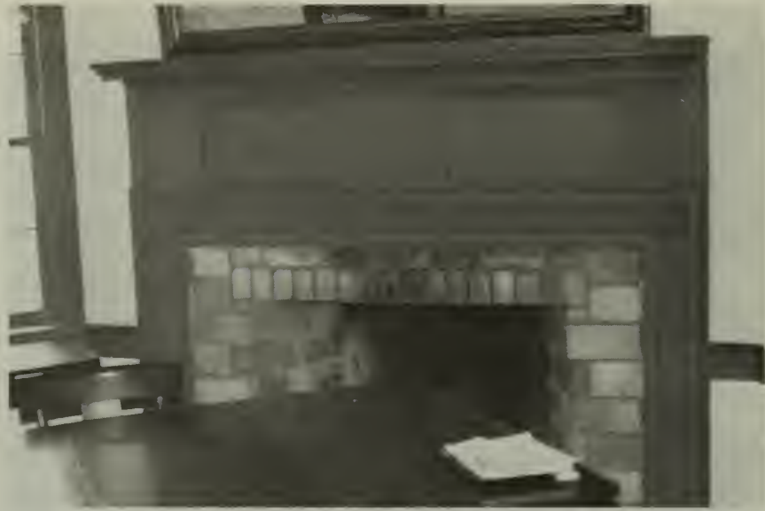
Southeast Corner - Room 105
