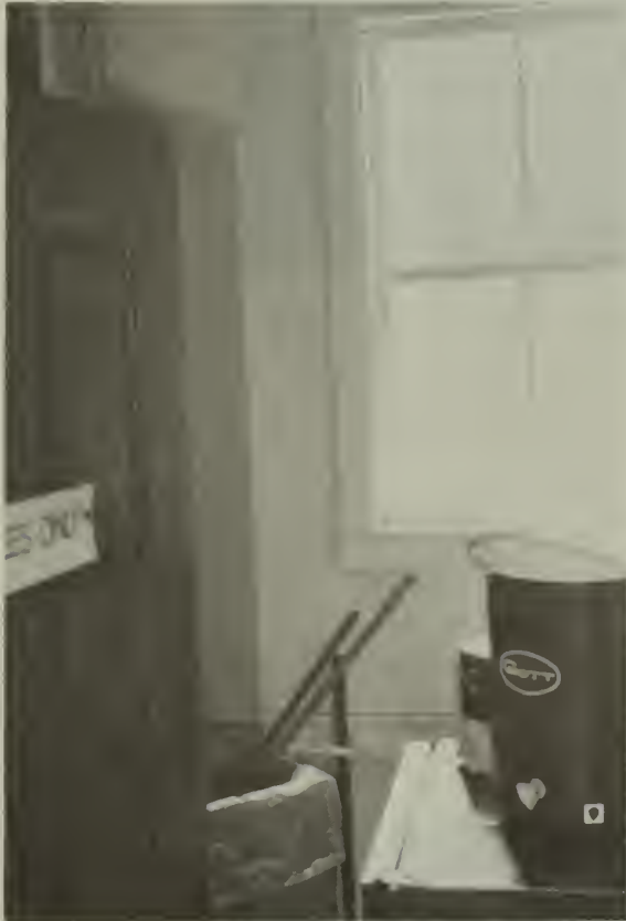
North Wall Room 205
