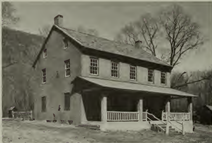
Slateford Farm Farmhouse - Front View
