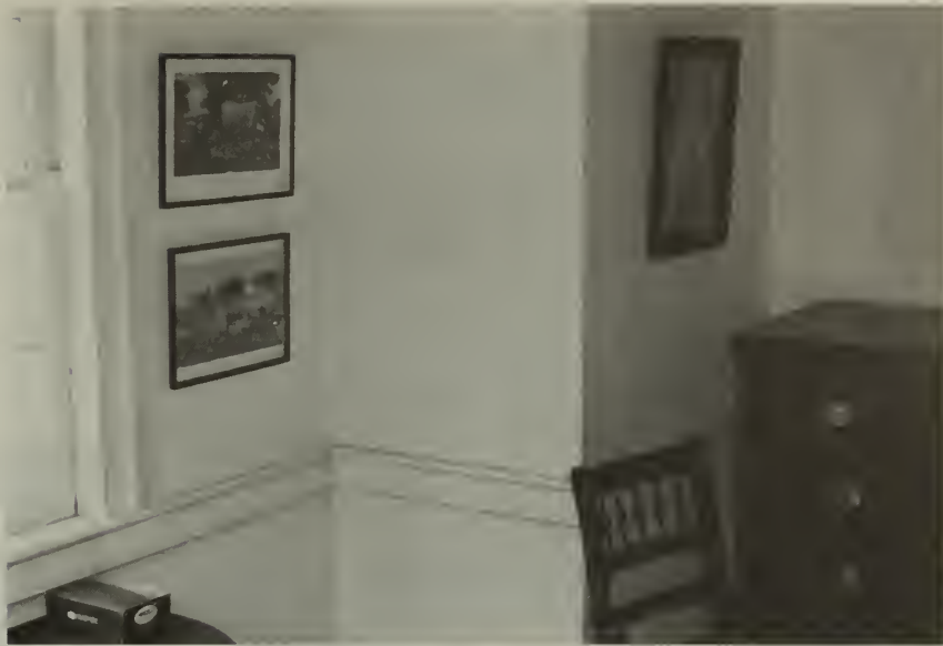
Southeast Corner - Room 206
