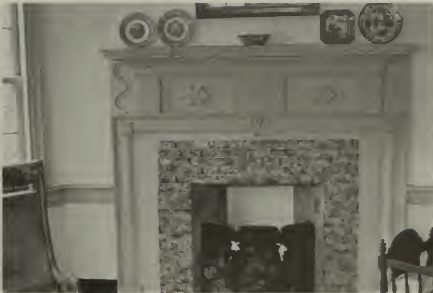
Northwest Corner - Room 203
