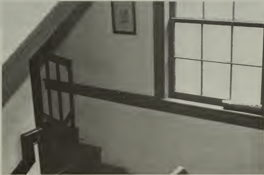
Center Stairwell, Looking Northwest - Room 201
