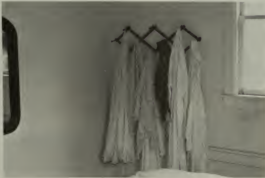
Northwest Corner - Room 206
