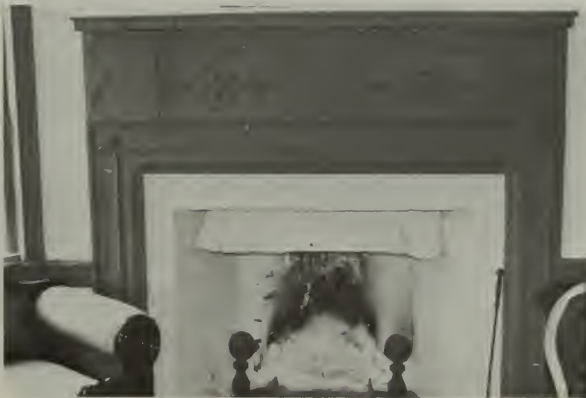
Northwest Corner Fireplace - Room 102
