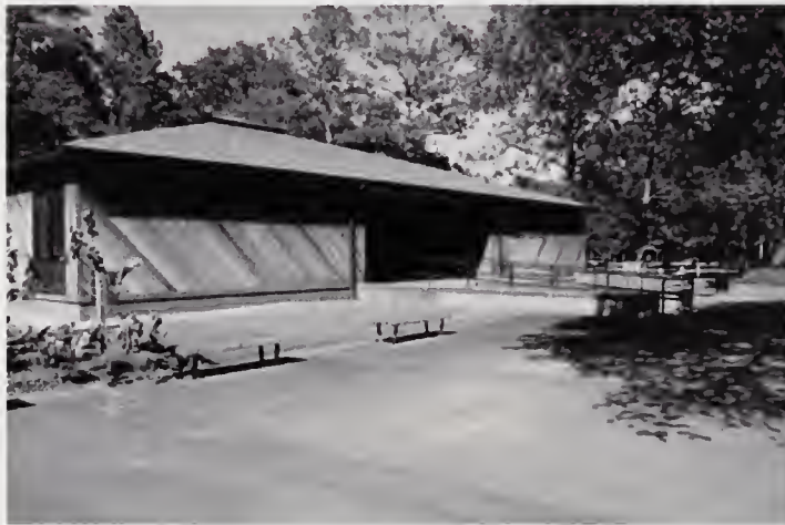
FIGURE 72. Wood and metal benches near the visitor center. Source: JMA, Inc., 2009.
