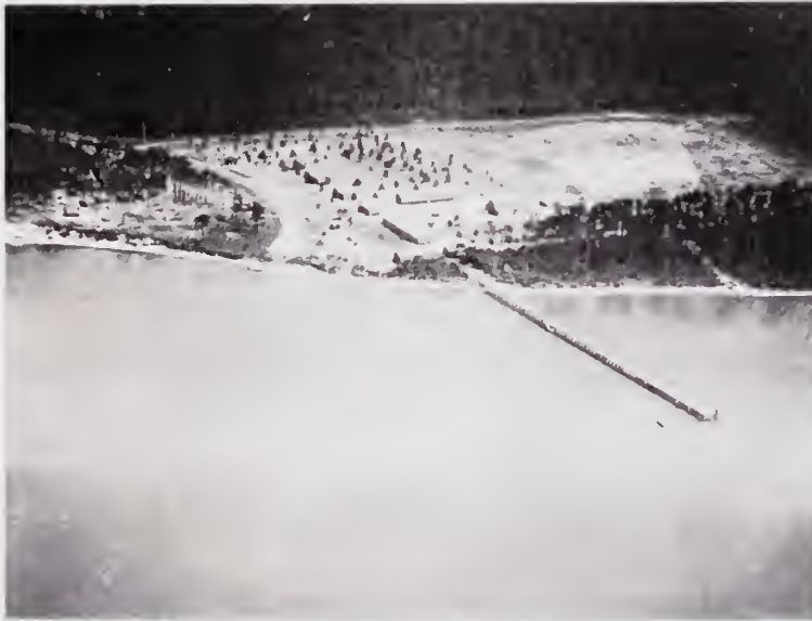
FIGURE 7. Camp Wirth, looking west-southwest. Source: National Archives.
