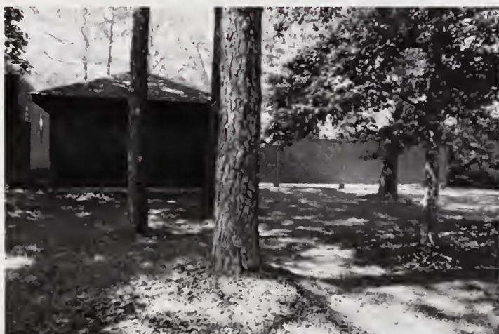
FIGURE 39. One of the generator buildings. Source: JMA, Inc., 2009.
