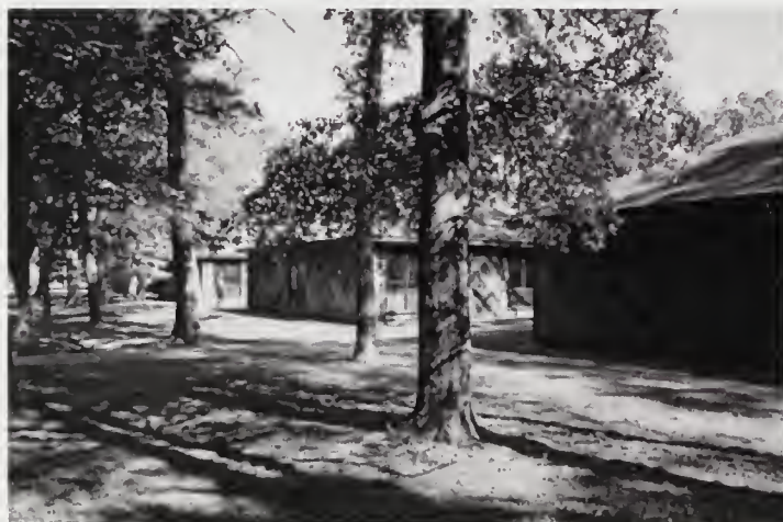
FIGURE 36. Outer Banks Group Support Office. Source: JMA, Inc., 2009.
