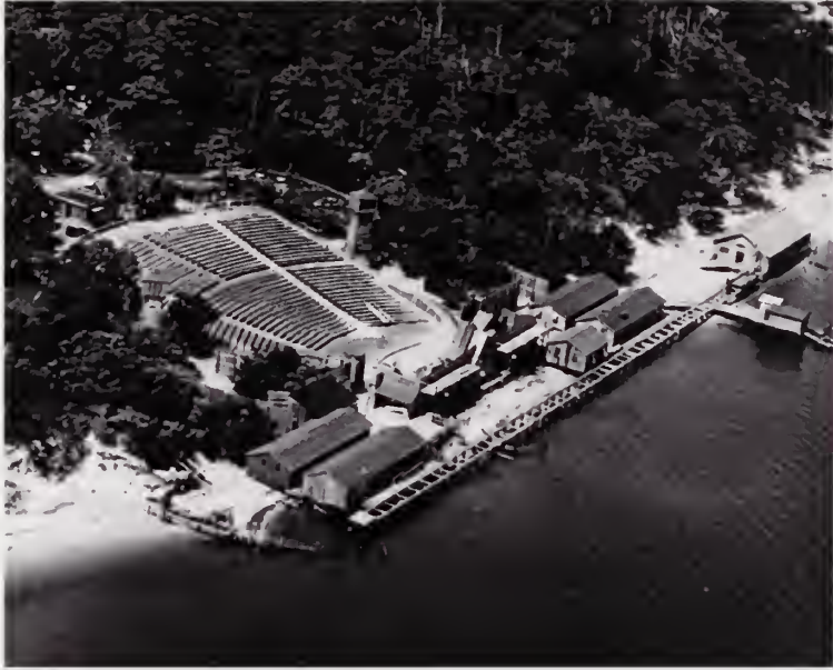
FIGURE 15. The Waterside Theatre, HABS photograph, HABS NC 389, undated.
