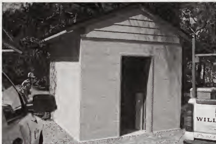
FIGURE 55. Lost Colony Storage Facility. Source: Fort Raleigh NHS, 2010.
