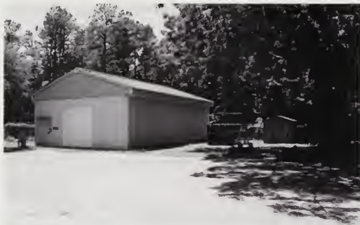
FIGURE 46. The Museum Resource Center Garage. Source: JMA, Inc., 2009.
