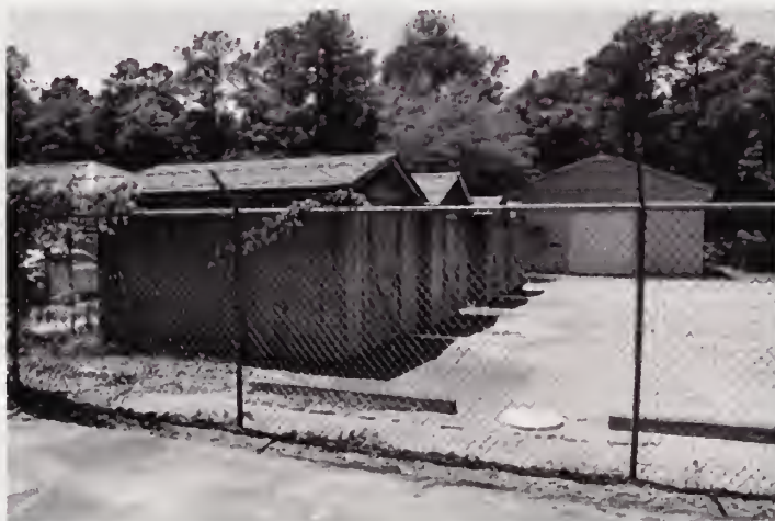
FIGURE 86. Chain link fence in the maintenance yard. Source: JMA, Inc., 2009.
