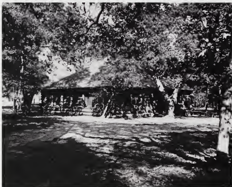
FIGURE 14. The visitor center, HABS photograph, HABS NC 389, undated.
