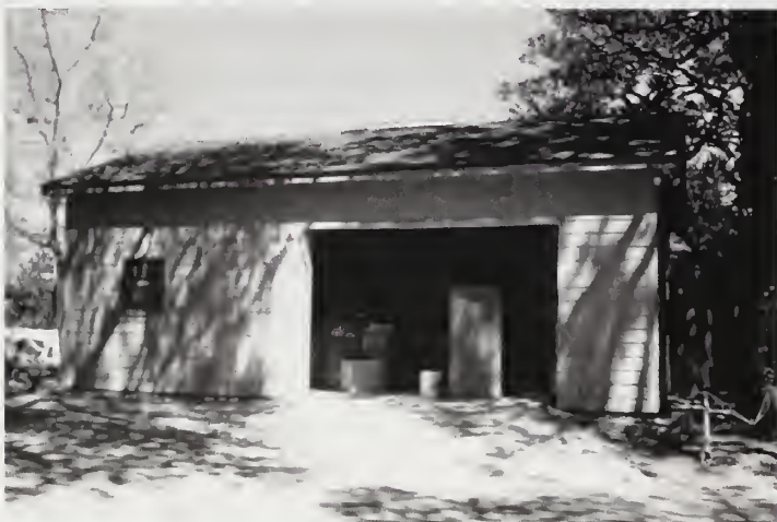
FIGURE 54. Lost Colony Maintenance Facility. Source: Fort Raleigh NHS, 2010.
