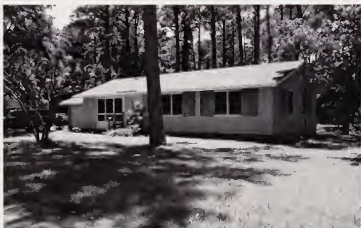
FIGURE 50. One of four small wood-frame residences. Source: JMA, Inc., 2009.
