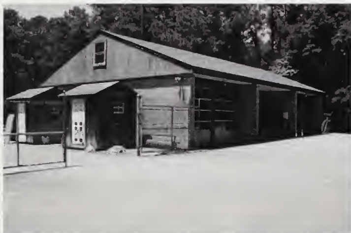
FIGURE 47. The Maintenance Building. Source: JMA, Inc., 2009.
