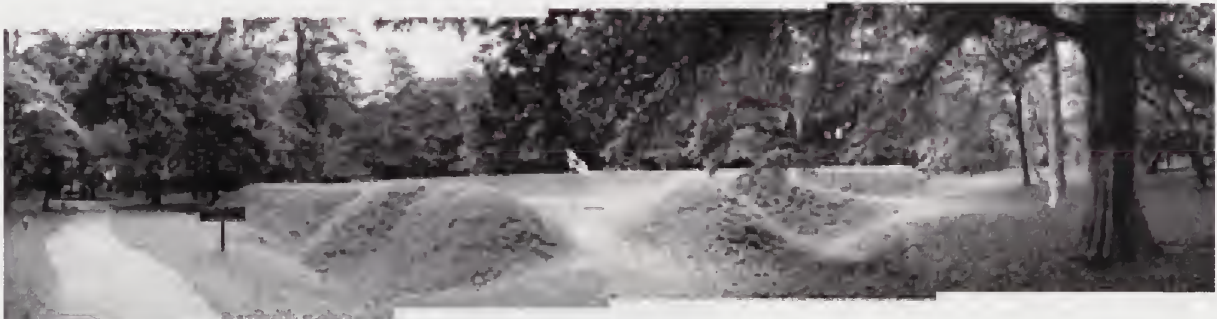
FIGURE 23. The earthwork fort, reconstructed in the 1950s. Source: WJE, 2009.
