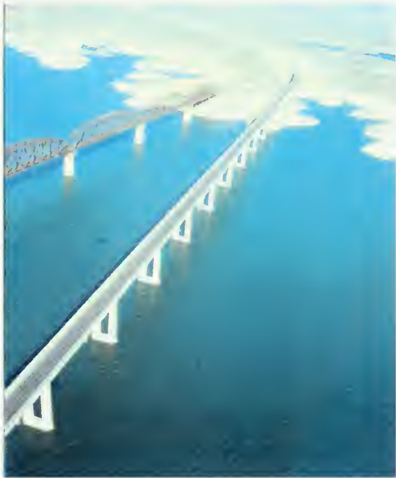
Figure 22. Railroad and Hwy 90 Bridges Crossing Amistad Reservoir
