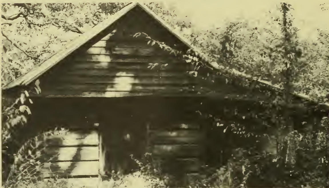
Old Farm Outbuilding
