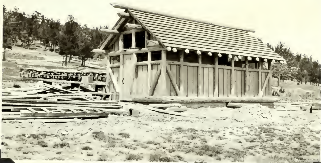
No. 13022-1. New comfort station, Mammoth Auto Camp, partly completed.
