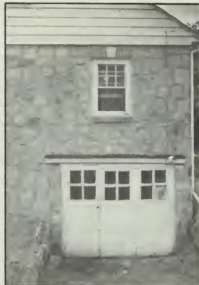
Figure 14 Garage built into basement.
