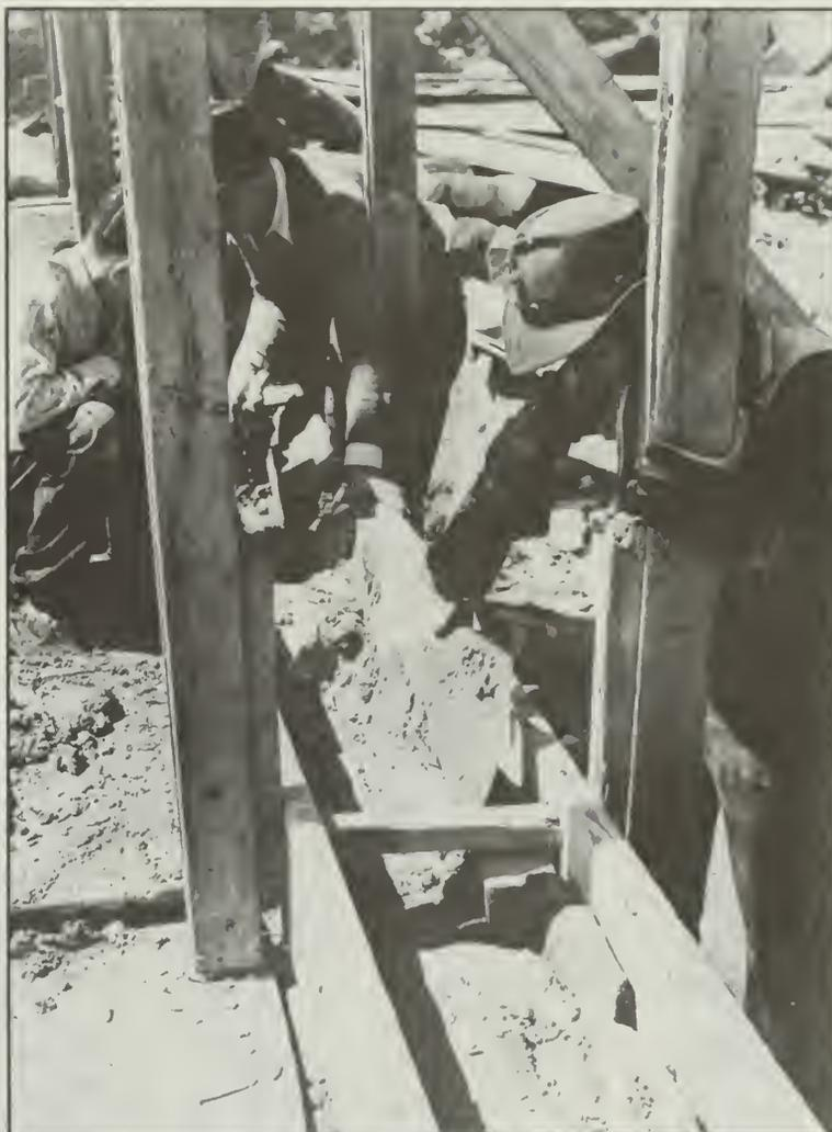
Figure 22 Forms used for construction of stone walls. Photographer unknown (1942), AFSC.
