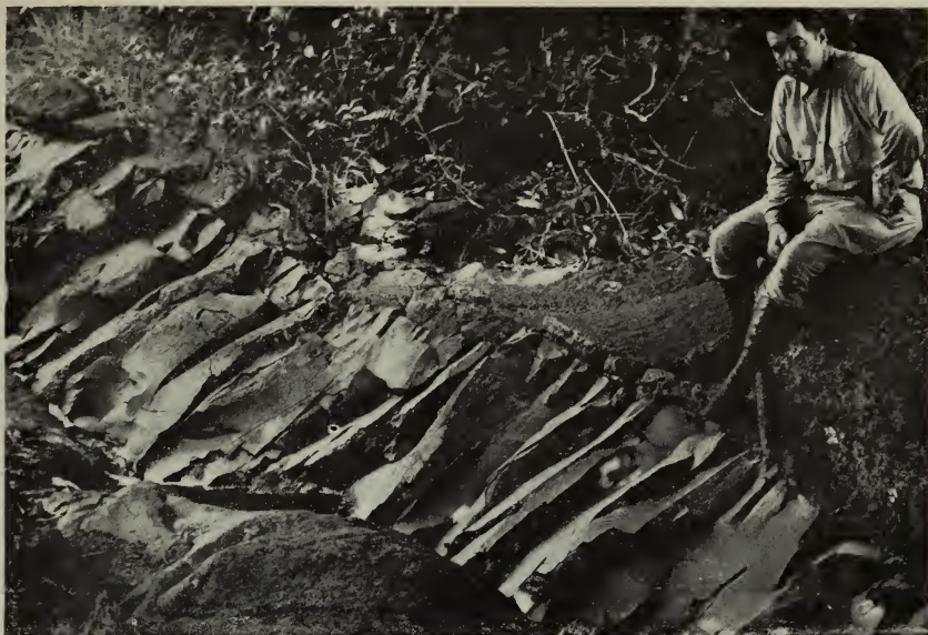
FIGURE 43.—Dike in channel of Wailupe Stream, Oahu, showing principal columnar jointing. Near the end of each column is splinter jointing that marks the dike margin. Photo by C. K. Wentworth.
