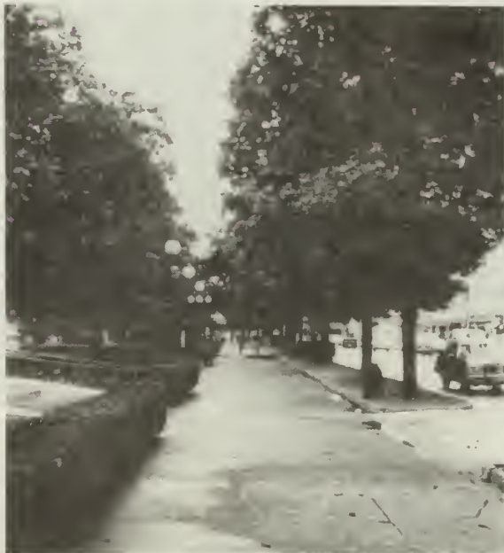
Figure 29. Magnolia Promenade Subunit, Looking South, 1984 (Source: Hot Springs National Park)
