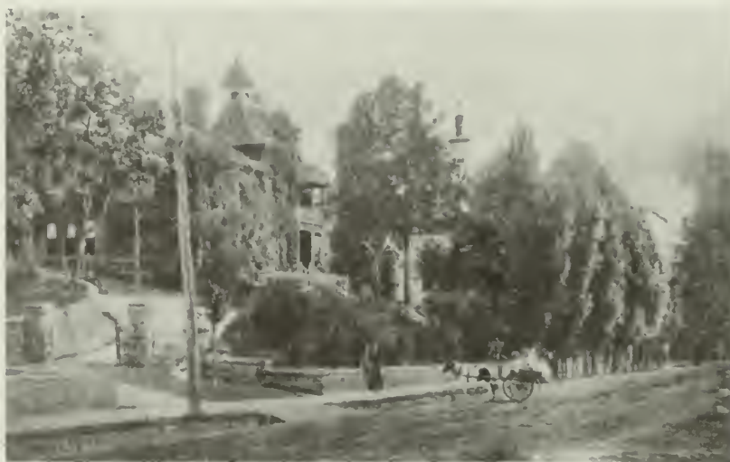
Figure 16. Superintendent's Residence, Fountain Street, ca. 1906 (Source: Hot Springs National Park)
