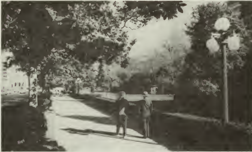
Figure 28. Magnolia Promenade Subunit, Looking North, 1984 (Source: Hot Springs National Park)
