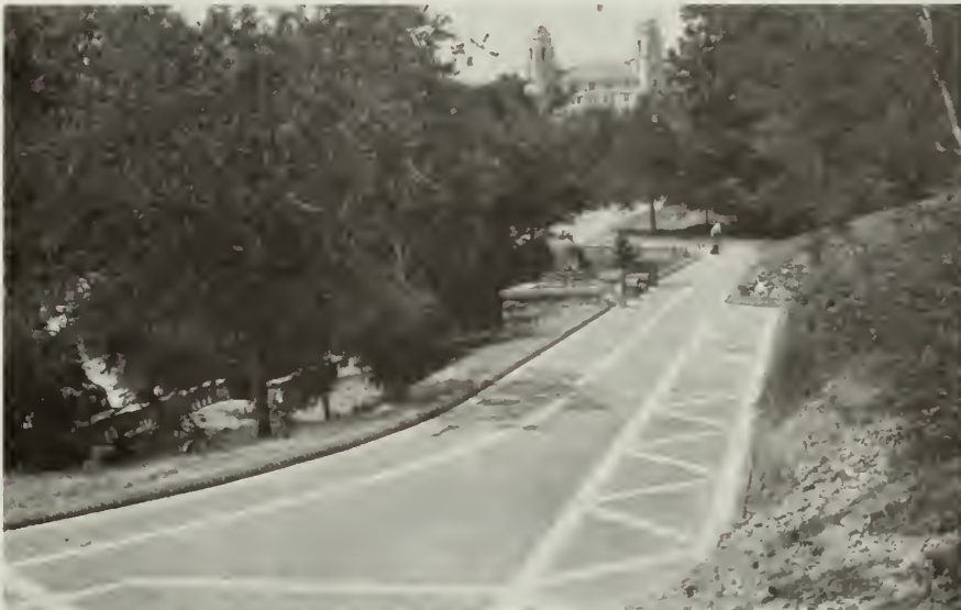
Figure 46. Grand Promenade Subunit, Looking North at Point where Main Entrance Ties into Promenade, date unknown (Source: Technical Information Center Photo Files, Denver Service Center, NPS, Denver)
