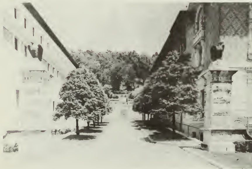
Figure 35. Main Entrance Subunit, Looking toward Stevens Balustrade and Grand Promenade, 1984 (Source: Historic American Buildings Survey)
