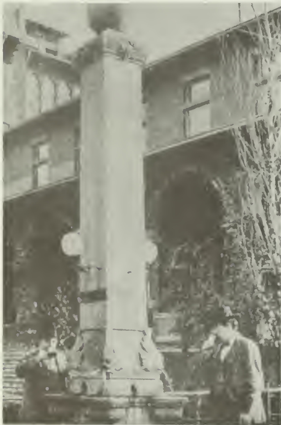
Figure 18. The Hoke Smith Fountain, date unknown (Source: Hot Springs National Park)
