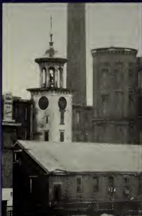
Boott Mills area before and after renovation.
