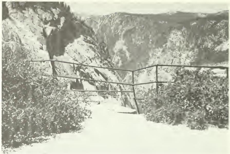
*Defective railing at overlook above precipitous cliff. Standards for location and maintenance are poor.*
