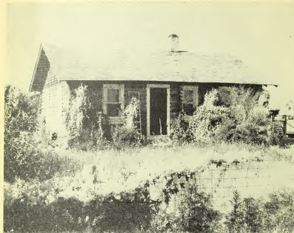
First year farm home, Riverton project, Wyoming
