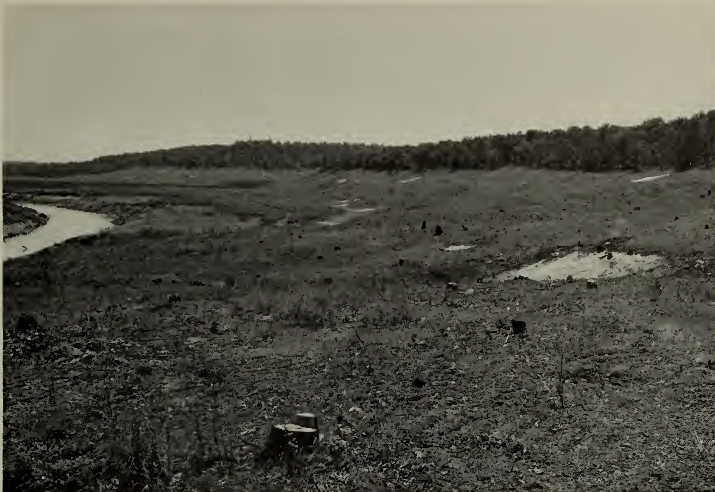
Figure 4.—Clearing (U. S. Engineer Office Photo)
