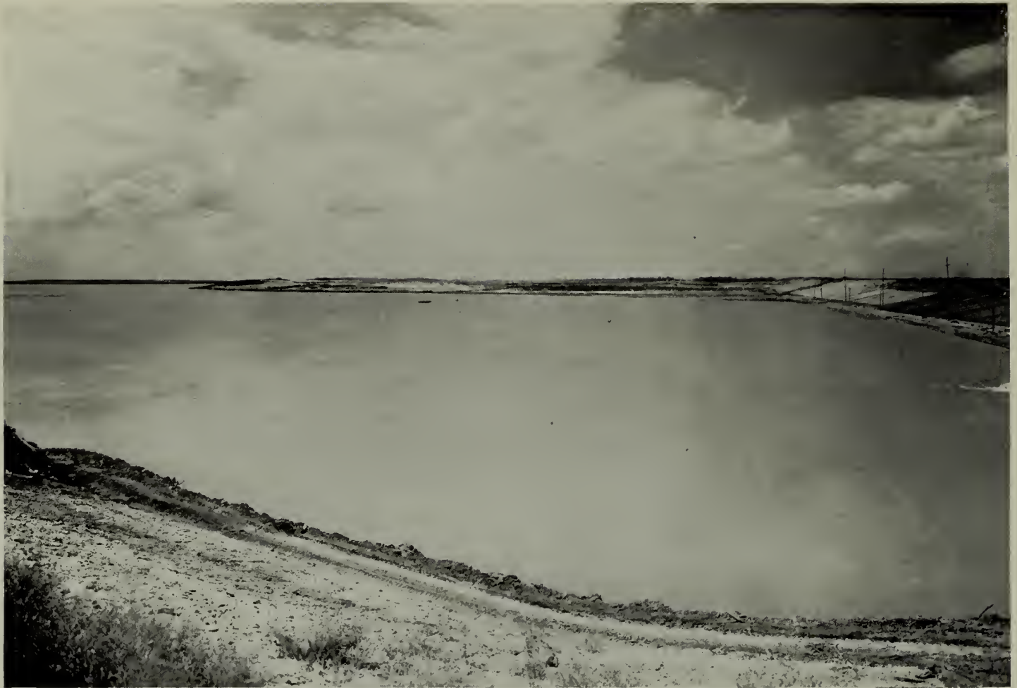
Figure 5.—Dam embankment (U. S. Engineer Office Photo).
