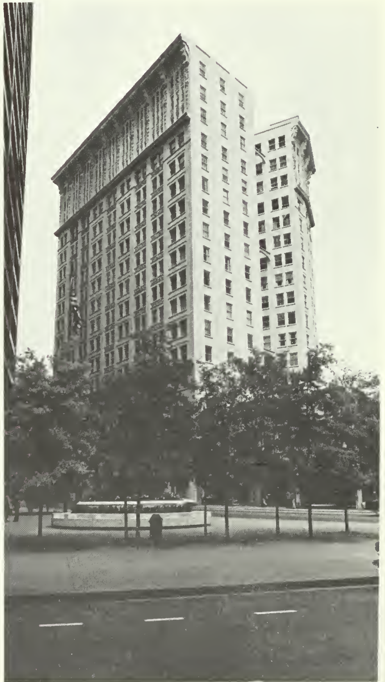
CANDLER BLDG. ATLANTA
