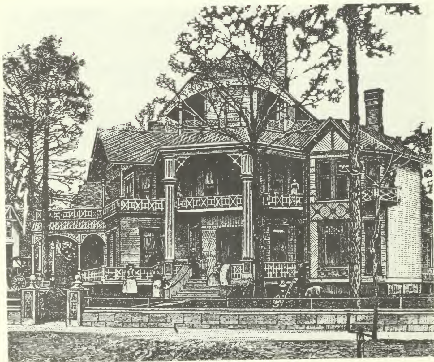
LAPHAM - PATTERSON HOUSE THOMASVILLE 1885 VIEW
