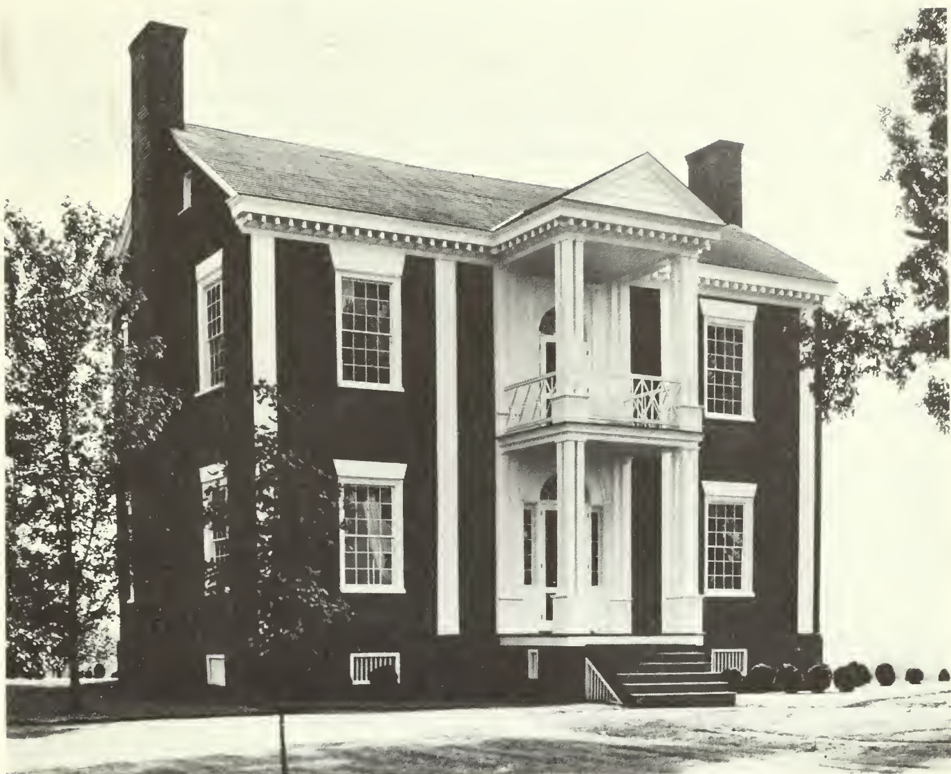
VANN HOUSE 1804 - SPRING PLACE
