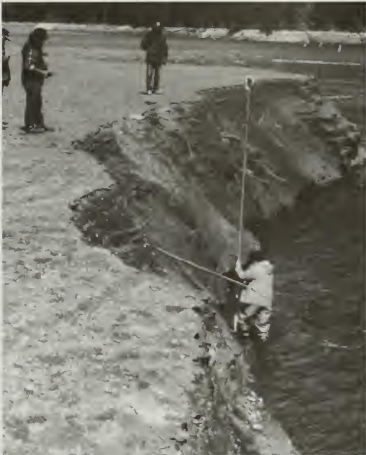
**Figure 18.** Land survey, with a total station and prism, of a Lake Mills Delta cross section.
