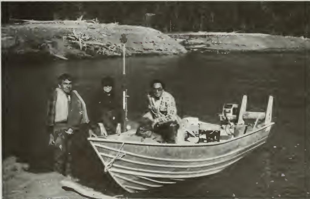
**Figure 19.** Bathymetric survey crew from the Lower Elwha Klallam Tribe and boat used to survey, with an electronic distance meter and fathometer, Lake Mills Delta cross sections that were too deep to wade.
