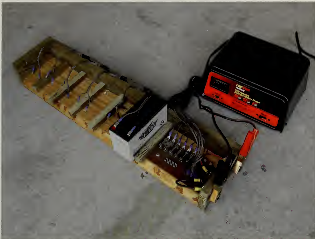
Figure 5. Example of a six battery bank charger. Each battery is individually fused to prevent catastrophic failure should an accidental short occur.
