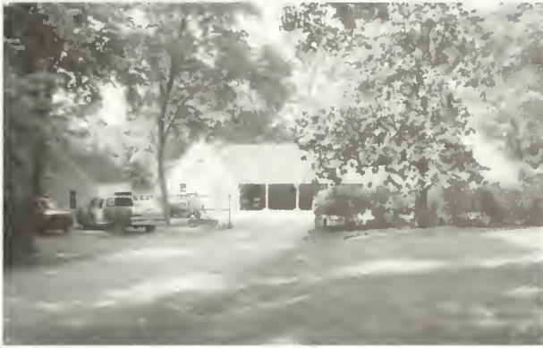
FIGURE 56. The Utility Building (Maintenance) and Inflammable Storage Unit.
