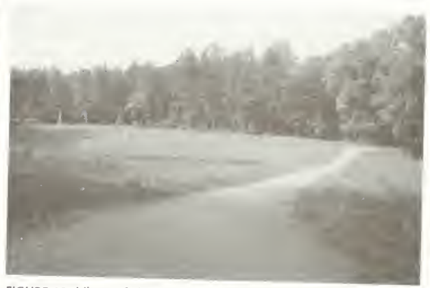
FIGURE 46. View of the New Garden trace exiting the woods, while traveling eastward, and traversing “Schenck’s field” (the field previously interpreted as the site of the third line), showing the Stuart Monument (left, middleground) and the taller Third Line Monument (far left, background).
