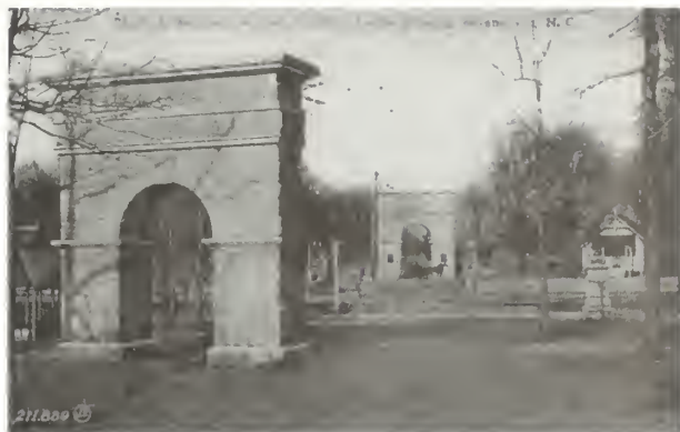
FIGURE 20. The Nash & Davidson Arches (erected 1905, dismantled 1937).
