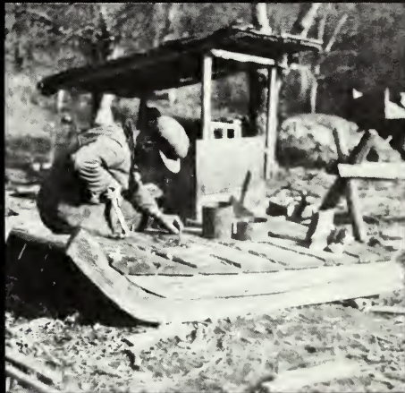
Repairing a hauling sled
