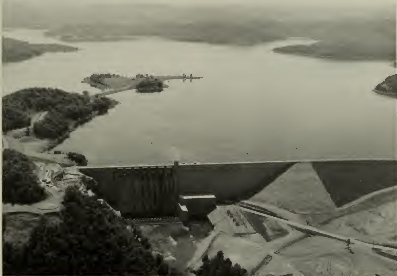
Beaver Reservoir is the uppermost reservoir on the White River system in northern Arkansas and southern Missouri. The conservation pool level is about 28,200 acres in area and has a storage capacity of about 1,650,000 acre feet. Depth at the dam is over 200 feet. (Photo by Sam Lanham)
