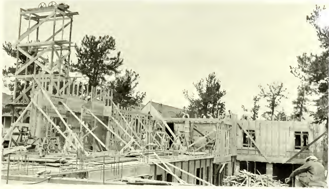
F.P. 346 - Apartment House, Mammoth (Pouring outside walls, North wing)
