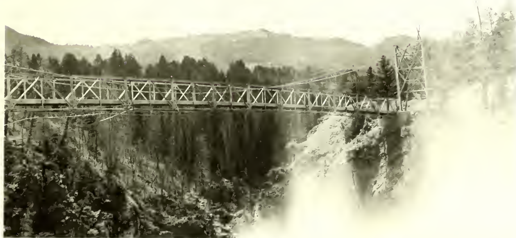
Project 509 - Elk Creek Suspension Bridge Bridge steel in place.
