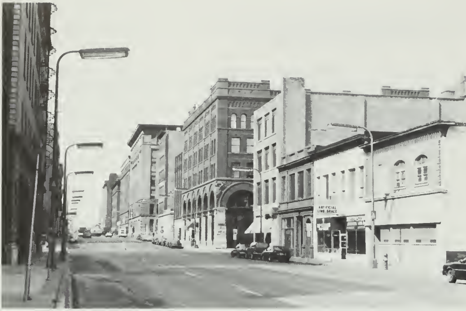
A streetscape in the Minneapolis Warehouse Historic District, Hennepin County, Minnesota, shows the diverse scale, period, and styles of the district's warehouses and commercial buildings. Begun as the city's warehouse and wholesaling center in the late 19th century, the district became a major shipping and jobbing center for the upper Midwest by the early 20th century. (Rolf T. Anderson)
