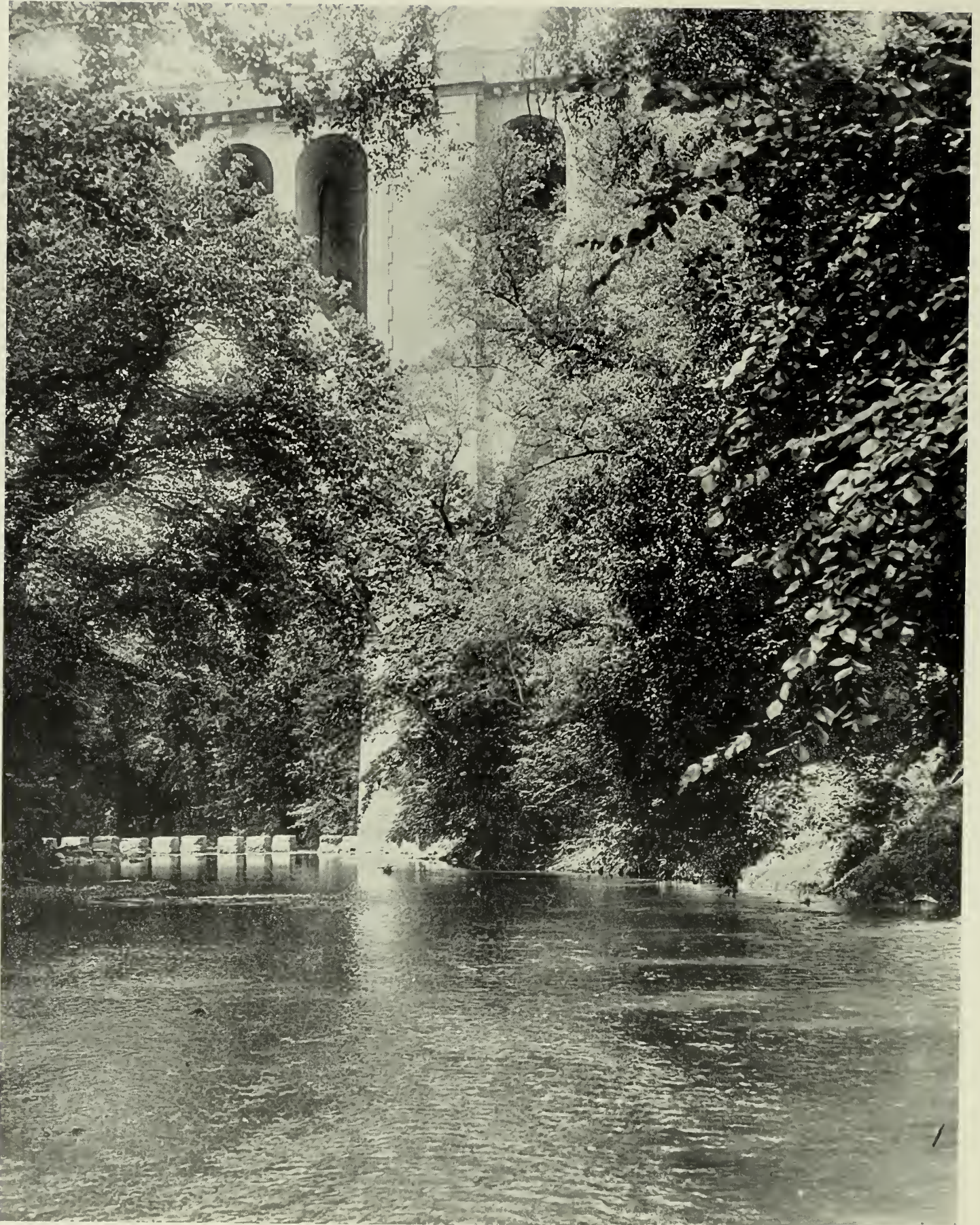
ROCK CREEK ABOVE CONNECTICUT AVENUE.
