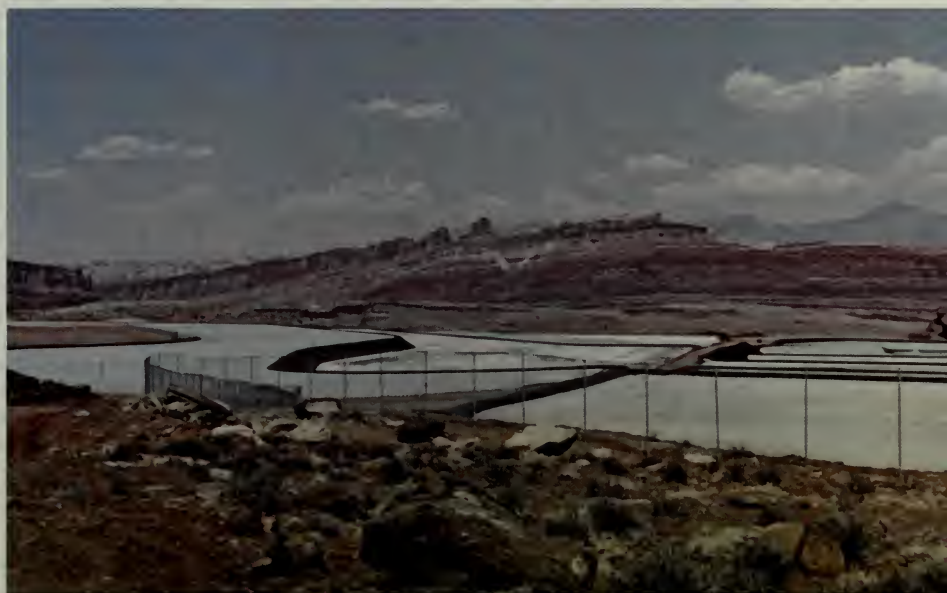
EVAPORATION PONDS, used to separate potash from common salt, viewed from jeep trail. Black borders are parts of plastic membranes covering bottoms of ponds. Crest of Cane Creek anticline and La Sal Mountains in right background. (Fig. 71)
