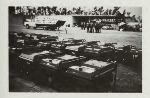
By early September, 200 small and 20 large generators were on the incident and capable of producing 2.2 megawatts of power. All critical facilities and power-dependent utility systems operated on generators from August 24 until commercial power was reconnected. This situation varied from September 21 at Everglades headquarters and Pine Island (when a temporary overhead line was installed) to early December for Flamingo when the new underground powerline was activated.
