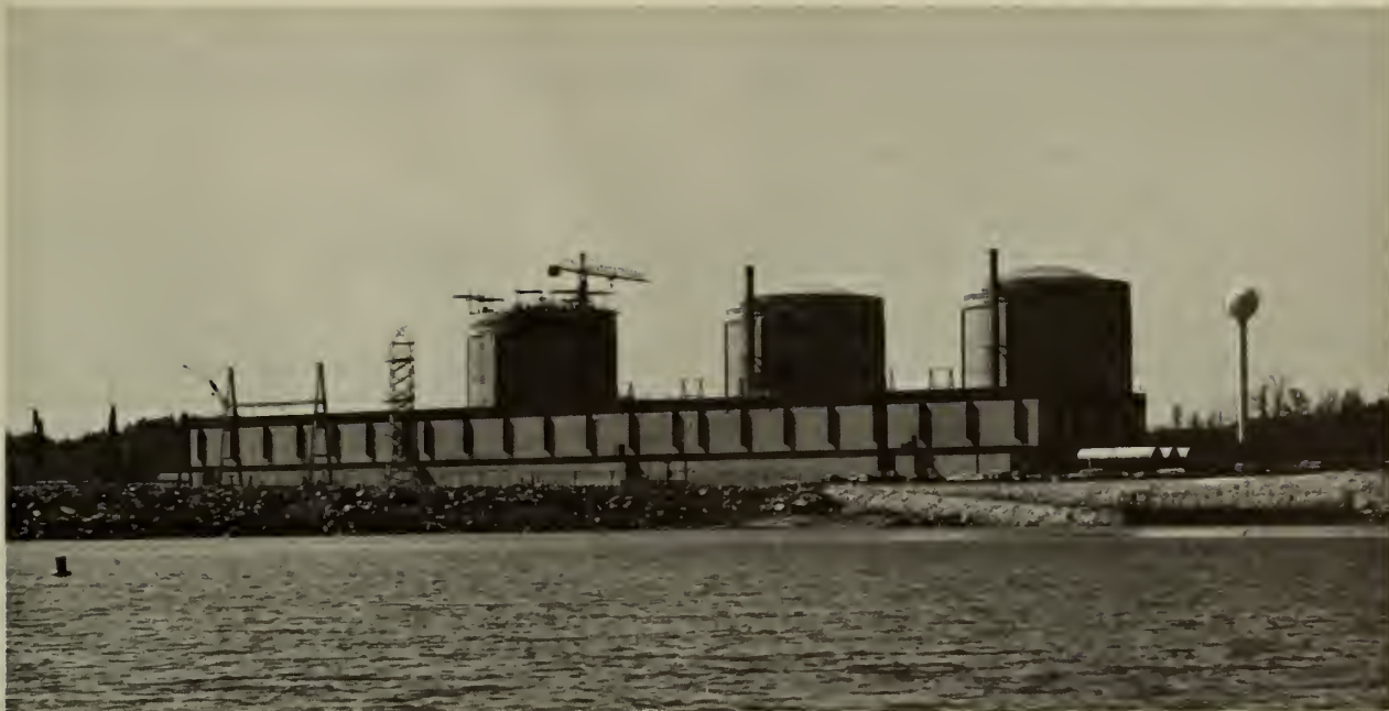
Duke Power Company's Oconee Nuclear Plant on Keowee Reservoir. About three-fifths of the energy produced from burning fossil fuels and two-thirds of that from the nuclear fission process at steam electrical generating stations are absorbed by condenser cooling water which is frequently discharged into the Nation's waterways. The Fish and Wildlife Service is conducting research to determine the effect of thermal additions to the aquatic environment (Southeast Reservoir Investigations photo)
