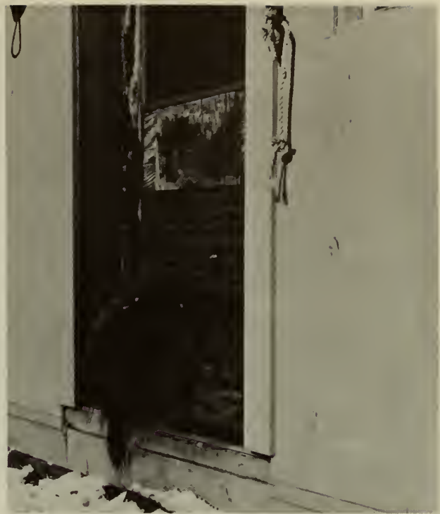
Porcupines cause thousands of dollars worth of damage annually to wood structures and signs. A cooperative study with the U.S. Forest Service determined which of 27 products tested were least susceptible to damage. (Photo by James Evans)
