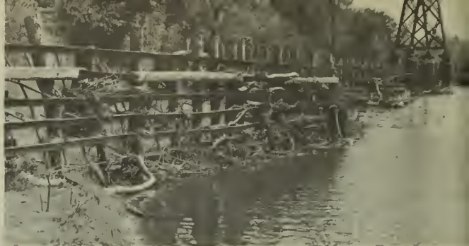
Metal and wood jetties used to protect bridge abutment on the Des Moines River, Iowa. Structure provides a scour hole and cover for fish even at low flow. Rock is superior as a construction material because it provides substrate for invertebrate production. Photo by R. V. Bulkley.
