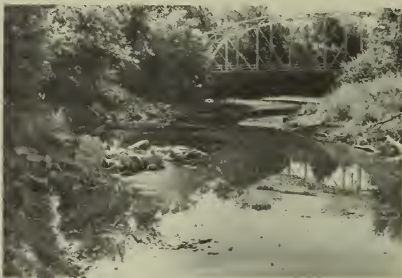
Rock jetties installed to protect a bridge provide shelter for fish on the Skunk River, Iowa, even at low-flow periods as shown here. In many streams with silt bottoms, these structures provide the major source of hard substrate for production of certain fish-food organisms. Photo by R. V. Bulkley.
