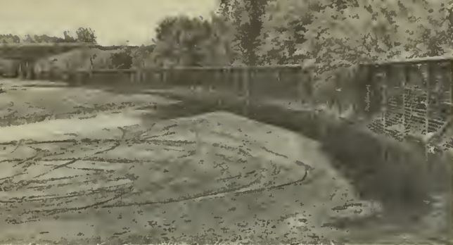
A bank stabilization structure. Even at low flow the structure, although not aesthetically beautiful, provides a scour hole at its base for fish shelter. Similar structures of rock are preferred from a fishery standpoint. Photo by R. V. Bulkley.
