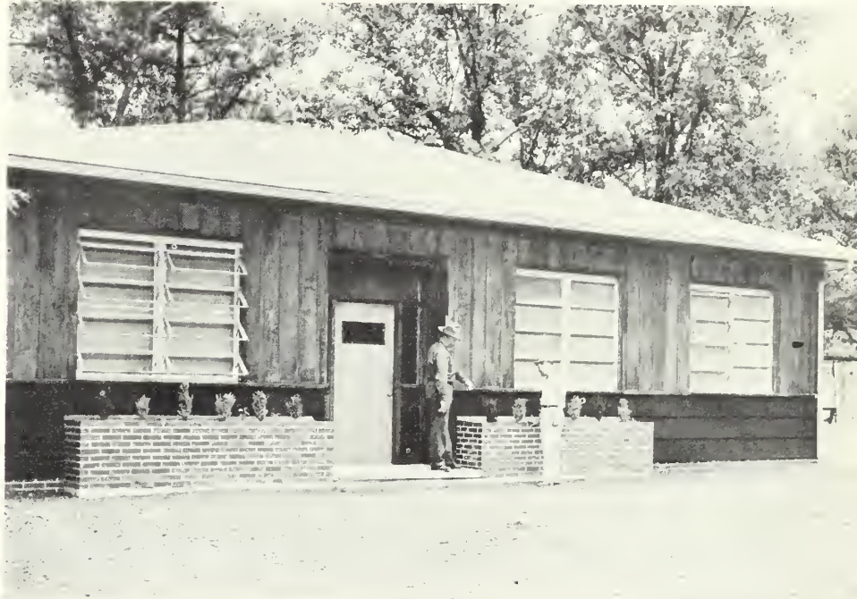
NEW HEADQUARTERS FOR WHITFIELD COUNTY FORESTRY UNIT--Commission personnel at Dalton are very proud of this modern building which will serve as their Forestry Unit headquarters.
