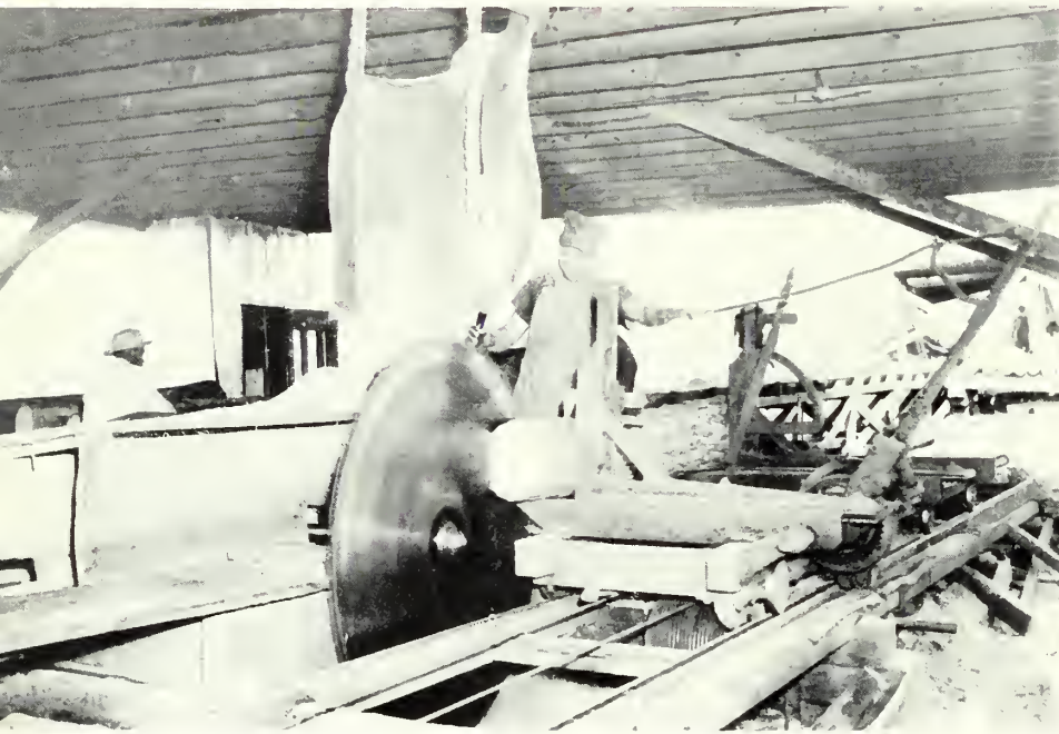
Logs are sawed into lumber (above). Lumber goes through planing mill (below).
