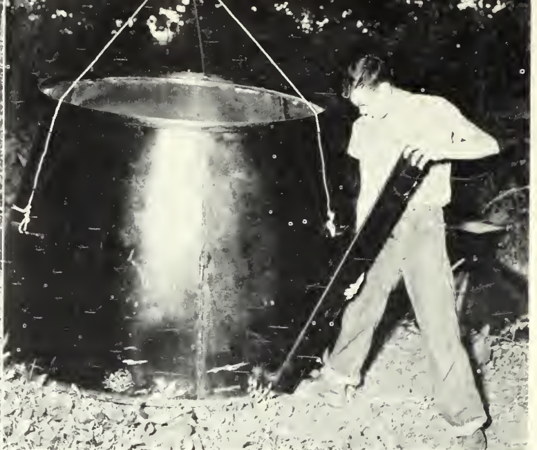
right photo Ware works with the kiln he uses to produce charcoal. He makes charcoal from small unmarketable hardwoods.
