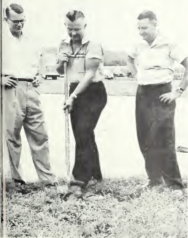
Albert drives corner stake; DeLoach breaks ground
