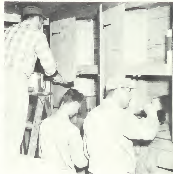
Management crew paints indoors, too
