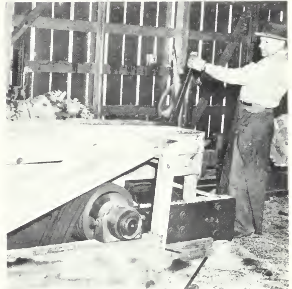
Gang saw cuts cant into boards
