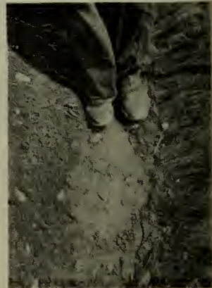
Tamp well; finish filling with soil.....
