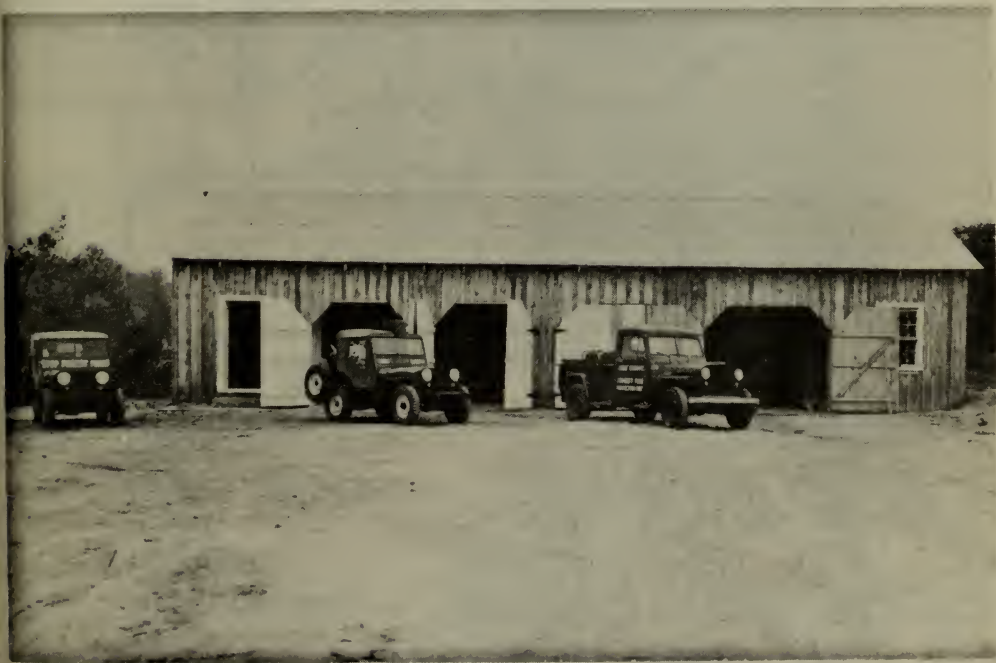
Pictured is the new headquarters of the Cobb County Forest Protection Unit at Marietta. Ranger Norman A. Medford has just moved his unit into the new building which provides officespace and adequate garage space for fire fighting vehicles.
