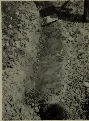
Dig sloping trench.....
