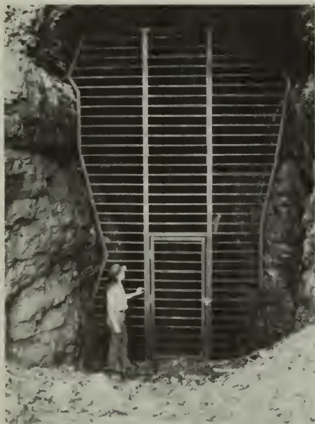
Natural Resource Specialist Margaret Weesner looks at a "bat gate" installed at the now reclaimed Kaymoor Mine. Photo by Margaret Weesner.
