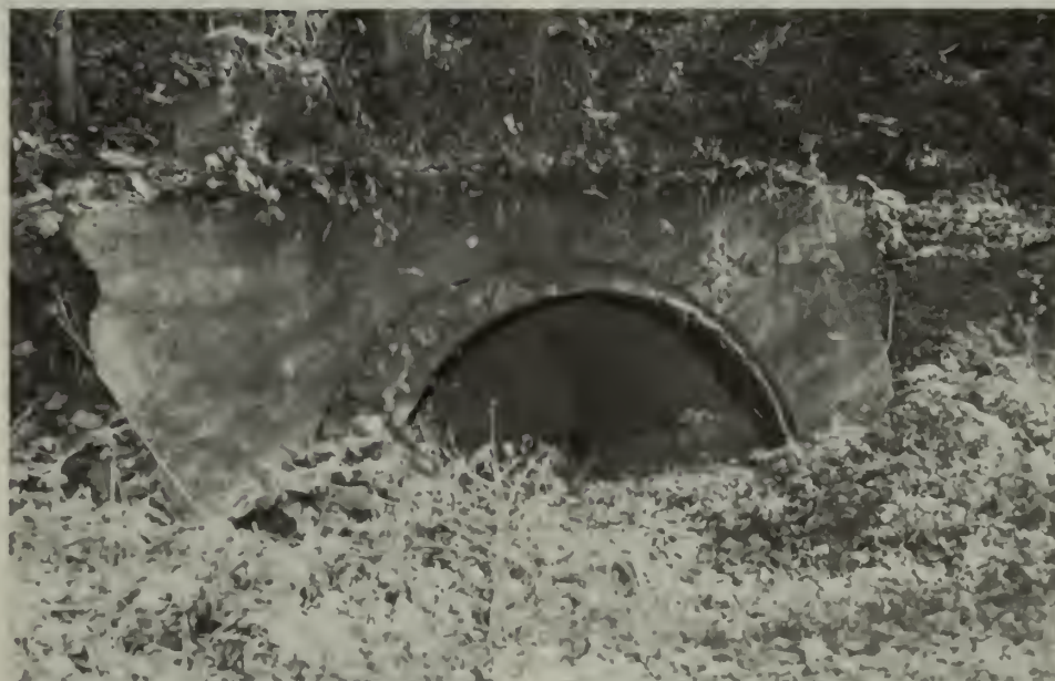
Open portal at Ames Mine. Photo by Robert Sullivan.
