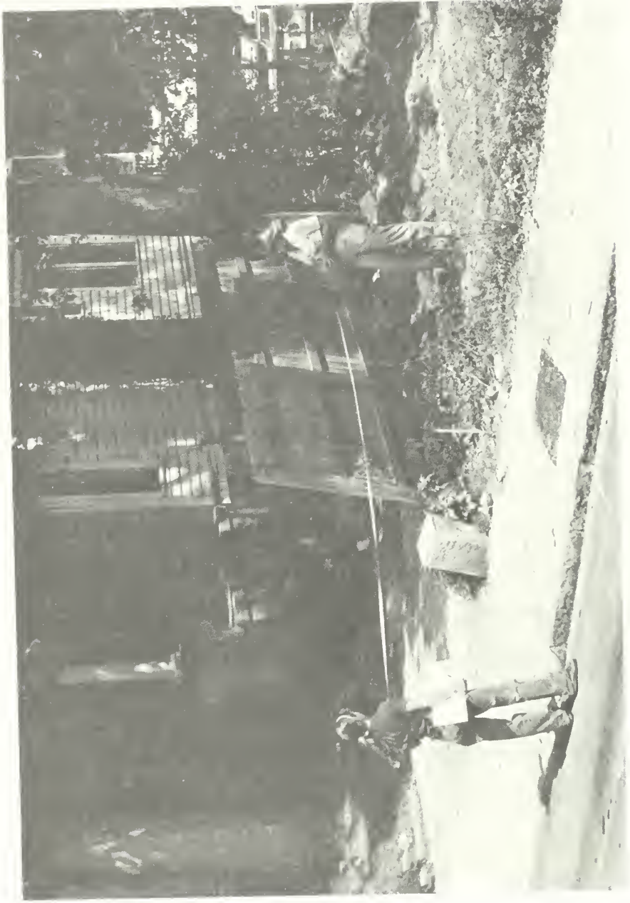
PLATE 1, DEFINING AN ARCHAEOLOGICAL SITE IN AN URBAN SITUATION BY TAKING MEASUREMENTS FROM A LOT CORNER MARKER, MARTA RAPID RAIL RIGHT-OF-WAY, ATLANTA.
