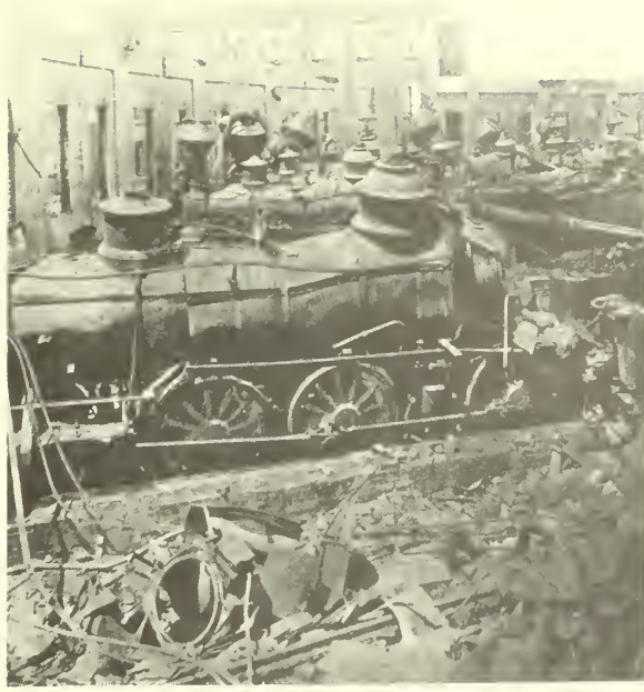
FIGURE 10: REMAINS OF THE LOWER ENGINE HOUSE, 26TH STREET, PITTSBURGH. Courtesy of the Pennsylvania State Archives, Harrisburg, PA.
