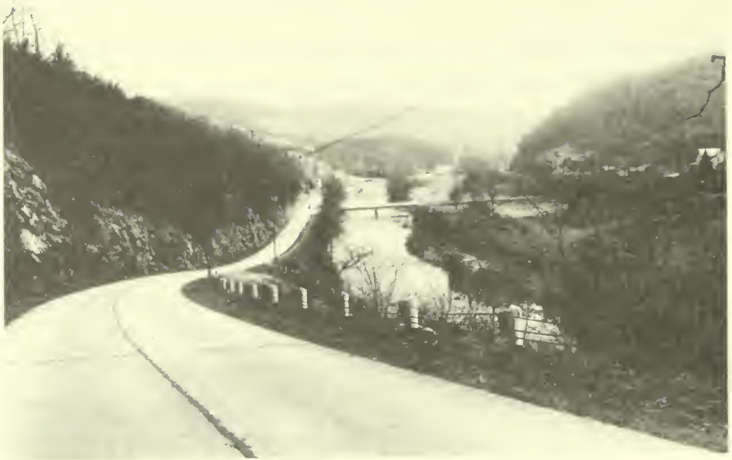
FIGURE 18: ROUTE #350 NEAR TYRONE, BLAIR COUNTY, PA. Early highway construction projects often fit the contours of the surrounding landscape, n.d. Courtesy of the Pennsylvania State Archives, Harrisburg, PA.
