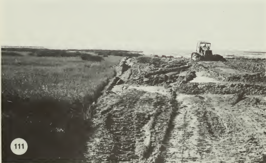
Fig. 111. Marsh adjacent to the same bay is being filled to make a parking lot for the boat launchers. This sort of thing would presumably not be done today.
