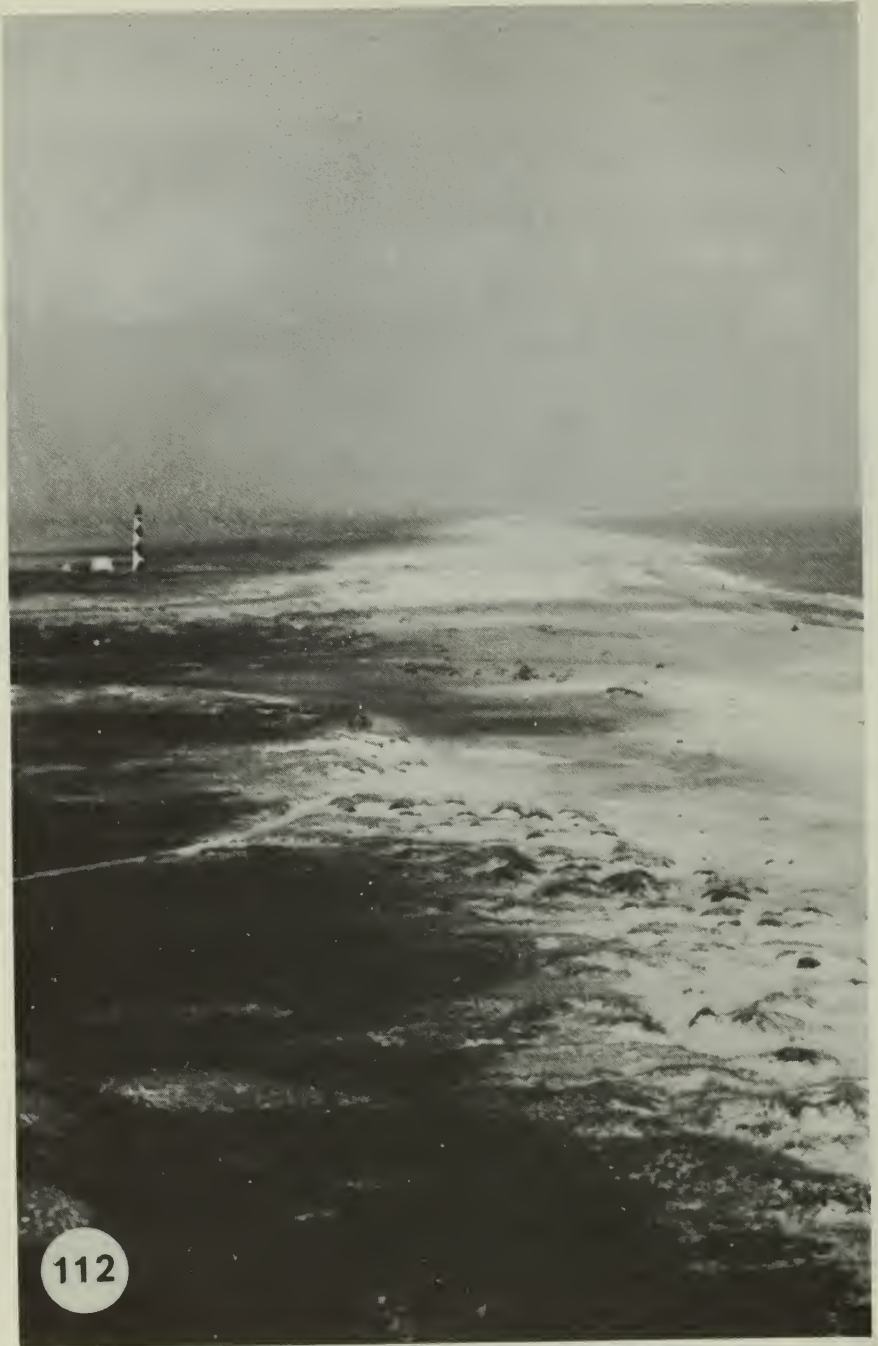
Fig. 112. Cape Lookout Lighthouse. Thirty or forty years ago the Hatteras Lighthouse was separated from the ocean by a similarly wide berm. (Photo by R. Simpson.)
