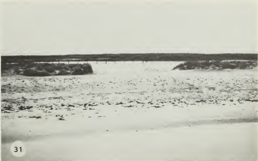
Fig. 31. The same storm drove water over the beach on Core Banks, with no damage except to experimental dune lines built with beachgrass on northern Core Banks; this straight dune line was continuous and storm surges piled up against it until a weak area broke through. Sand from the dune line was spread out in back as an overwash fan.
