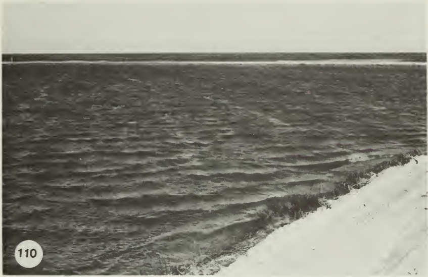
Fig. 110. This boat-launching bay was made by excavating a salt marsh to get fill to shore up an eroding dune line. Cape Hatteras National Seashore is in the background. The already vulnerable island has been further narrowed.
