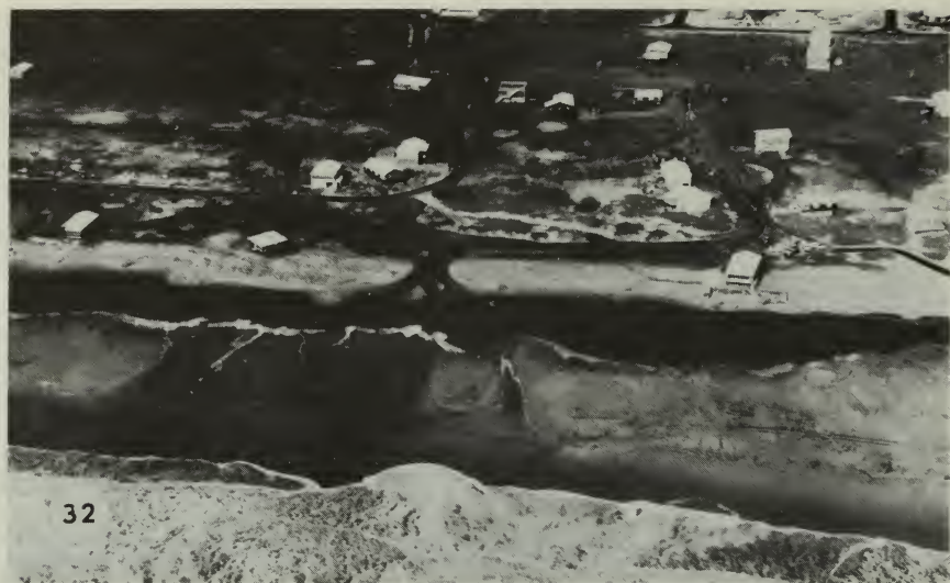
Fig. 32. Dune breaks and overwash caused considerable damage to cottages built too close to the beach. A storm on 28 March 1971 broke over the low dunes at Avon, a town within the boundaries of Cape Hatteras National Seashore, causing what is generally termed damage, although it was a predictable and natural event. (Photo by Cape Hatteras National Seashore Staff.)
