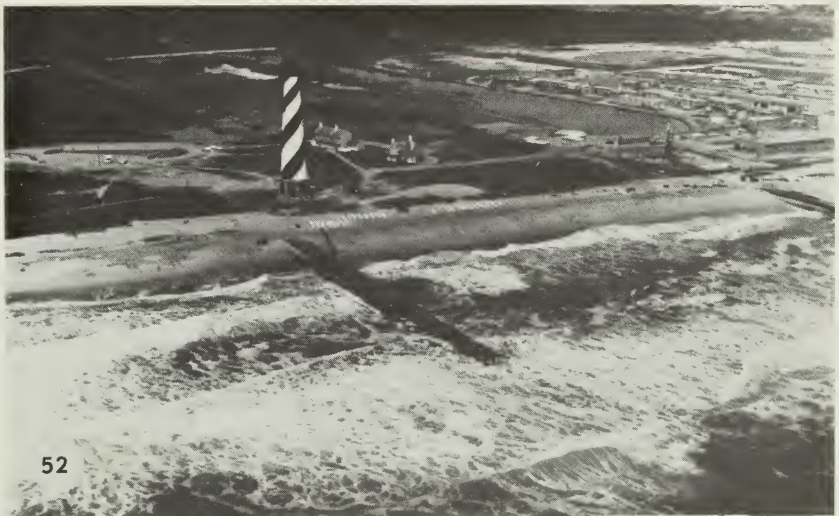
Fig. 52. The location of Cape Hatteras Lighthouse contrasts sharply with Cape Lookout. When this photo was taken 17 April 1970, the berm was non-existent. Groins under construction later caught sand, but caused other problems down drift. Storm waters are stopped at the dune line. In recent years much effort and money have been expended to keep the lighthouse from falling into the Atlantic Ocean. At Cape Lookout nothing at all has been done, yet that lighthouse is safe for the foreseeable future. The artificial dune line clearly exacerbates the erosion problem. (See Dolan in press.) (Photo by Cape Hatteras National Seashore Staff.)
