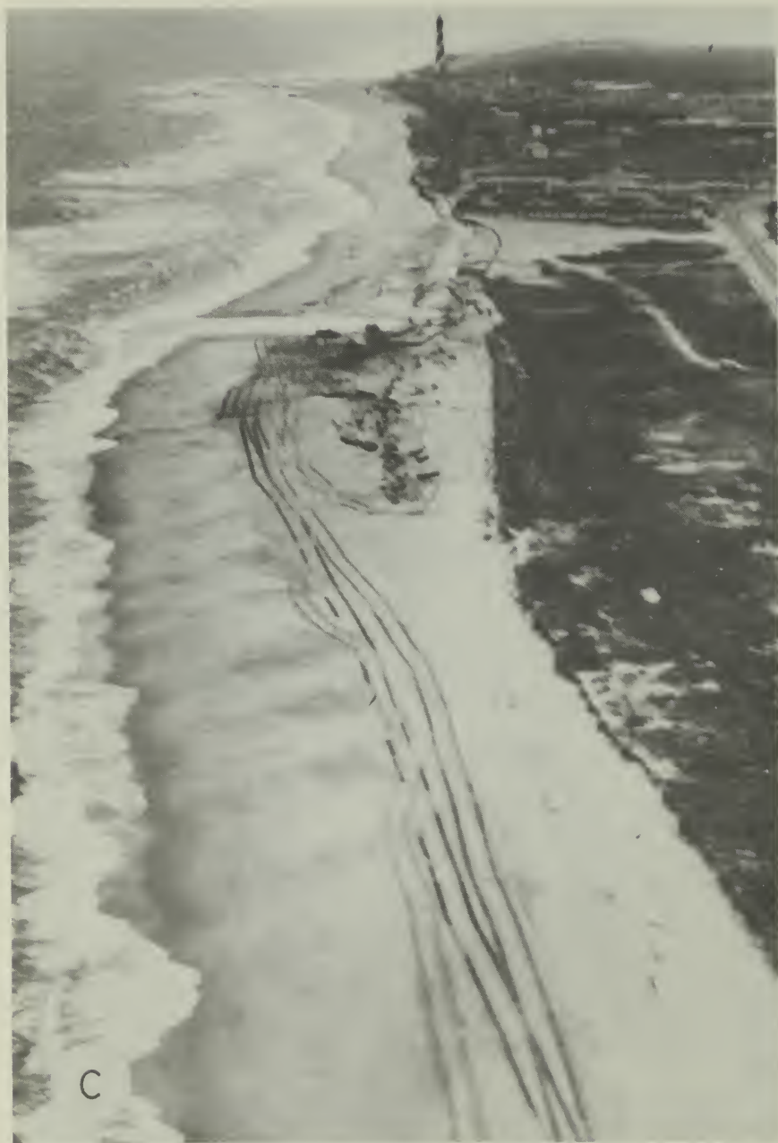
hold back the sea. ( Photo by Cape Hatteras National Seashore. ) (C) To remedy the situation in B, an experimental beach nourishment project was begun in February 1972, with sand pumped from Hatteras Point. The erosion problem in front of the motels is temporarily relieved. ( Photo by Cape Hatteras National Seashore. )
