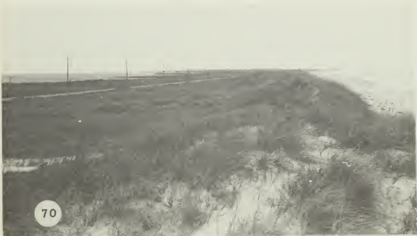
Fig. 70. Continuous man-made stabilized dune on Hatteras Island, eroding on the seaward side. The American beachgrass is very dense due to heavy fertilization. The great density of vegetation on these man-made dunes is a distinctive feature of such stabilization programs and is not normally seen on natural dunes. There are few other species and no sand movement back of the dunes. Open areas in the grass are caused by disease and insect attacks. In such open areas, sea oats becomes established and lends a more natural appearance to the dunes.
